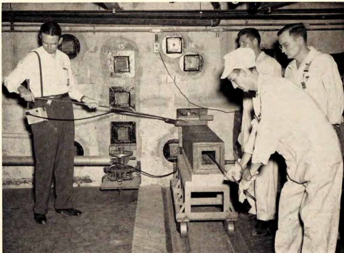
Figure 16. ABOVE: Pulling an isotope stringer from the atomic pile
