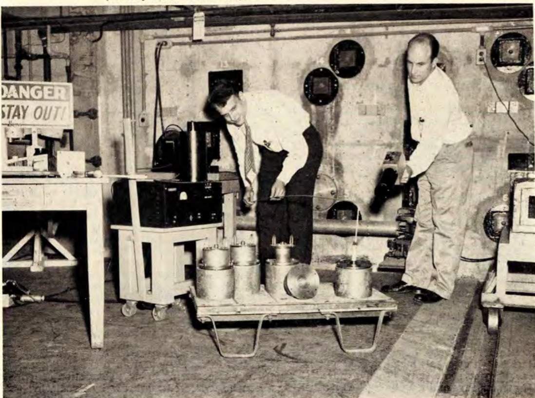
Figure 17. BELOW: Putting a can of radioisotopes in a lead shipping container (Courtesy United States Army)
