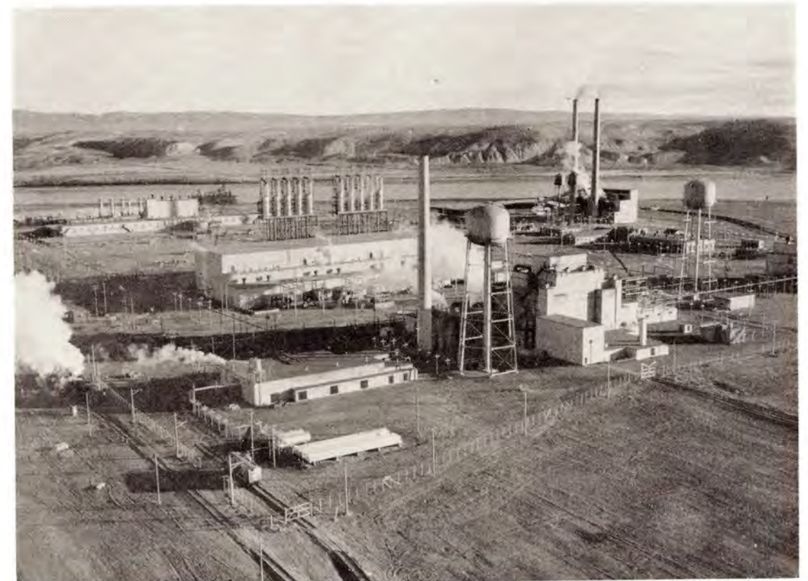
Atomic Energy Plant At Hanford, Washington (Courtesy Atomic Energy Commission)
