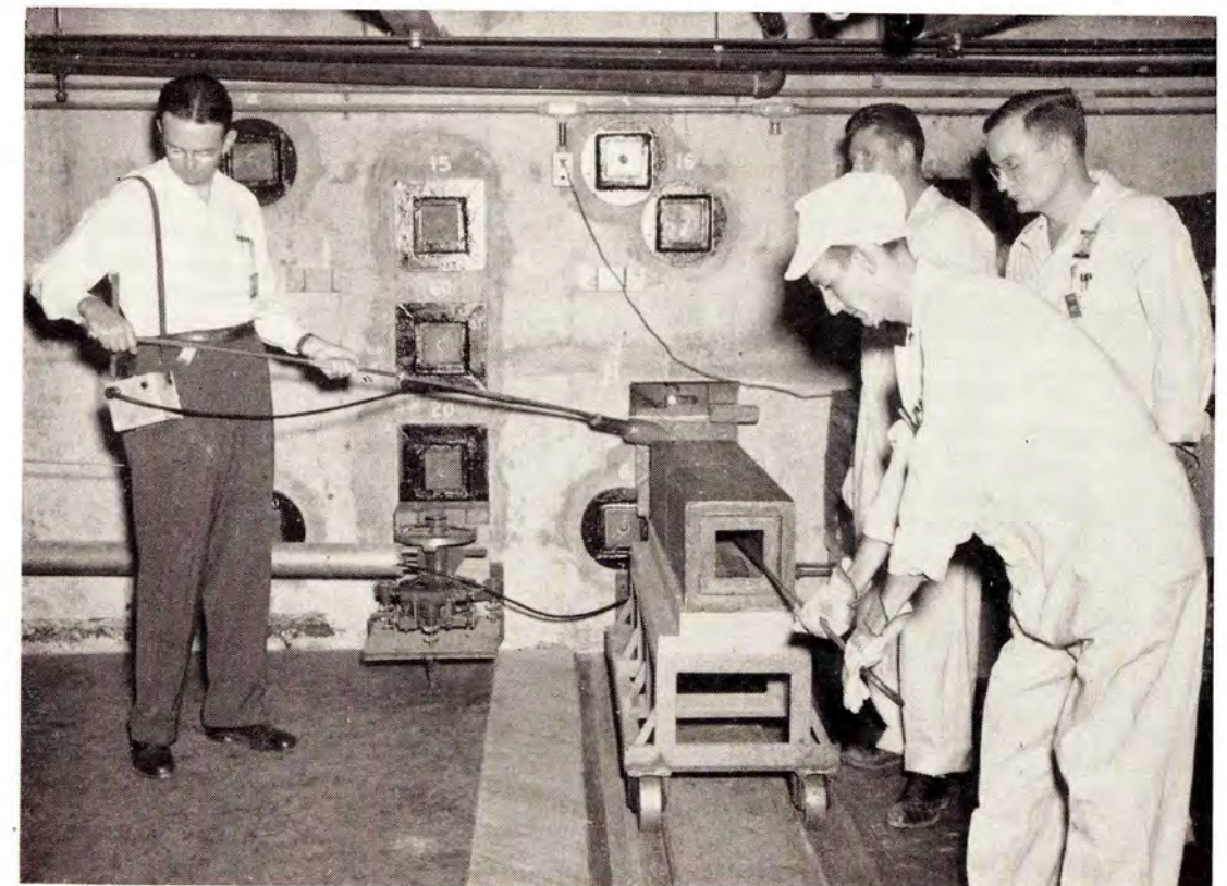
ABOVE: Removing isotopes from the atomic pile BELOW: Putting radioisotopes in a lead shipping container (Courtesy United States Army)
