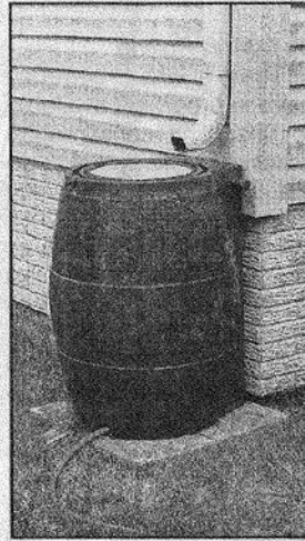
Rain barrels capture rainwater from downspouts and contain it for future use.
