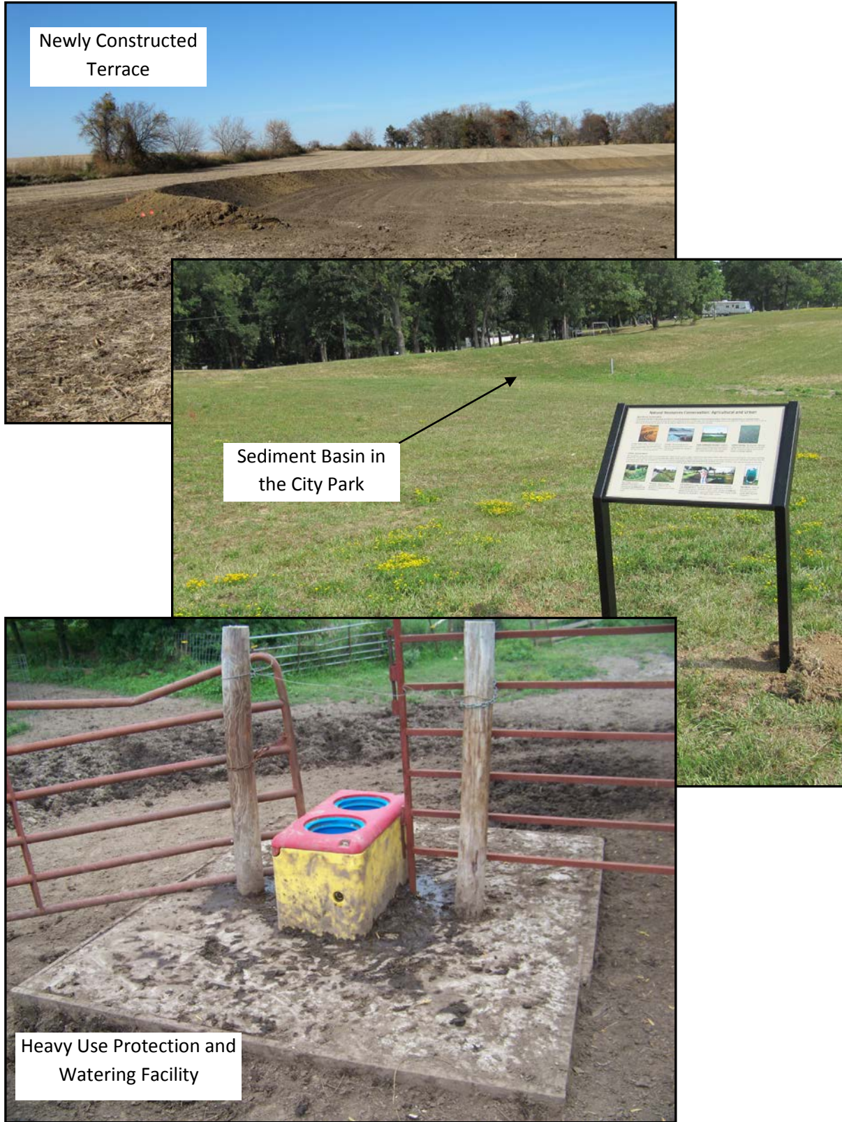
Figure 4. Photos of a new terrace, a sediment basin after the seeding has come in, and a heavy use protection and watering facility associated with a rotational grazing system.
