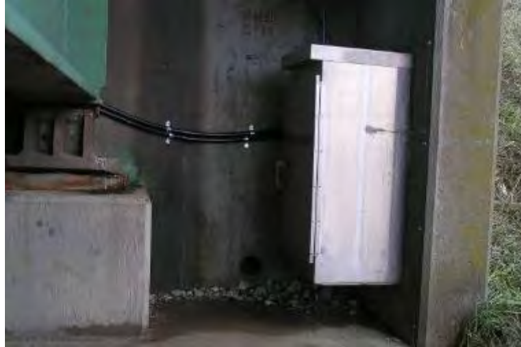
(a) Aluminum cabinet mounted on the north corner of the west abutment wing wall
