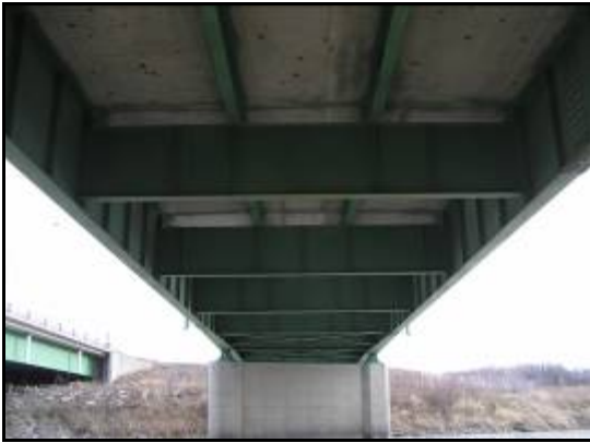
b. Girders, stringers, floor beams, and stiffeners
