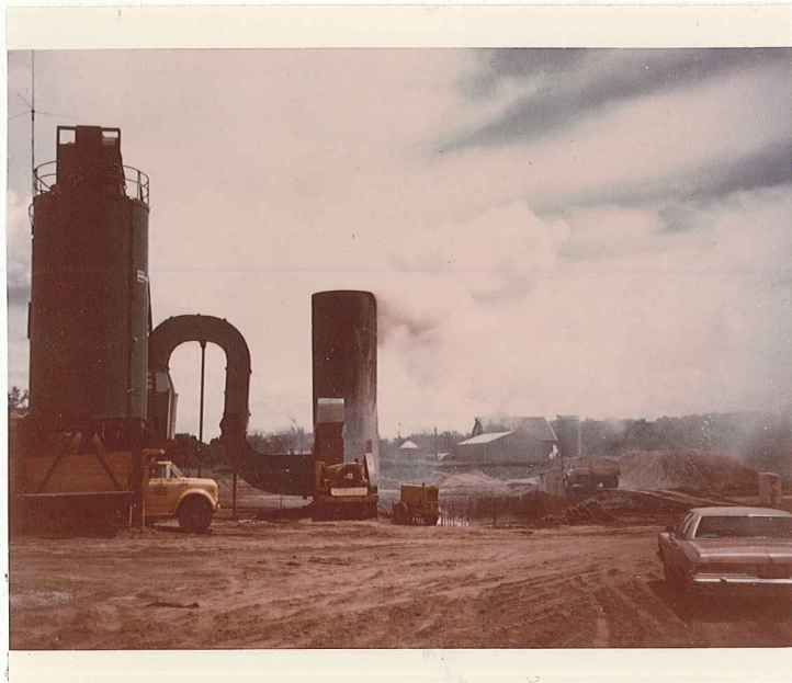
Production - using 3% moisture, wet wash, lower temperature, and lower production. Note blue haze.
