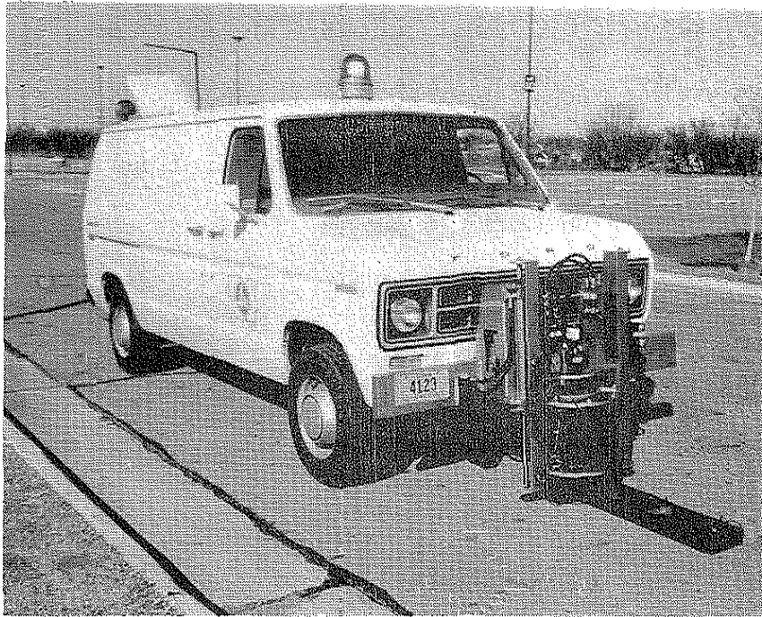
Figure 5. Road Rater as Originally Front Mounted
