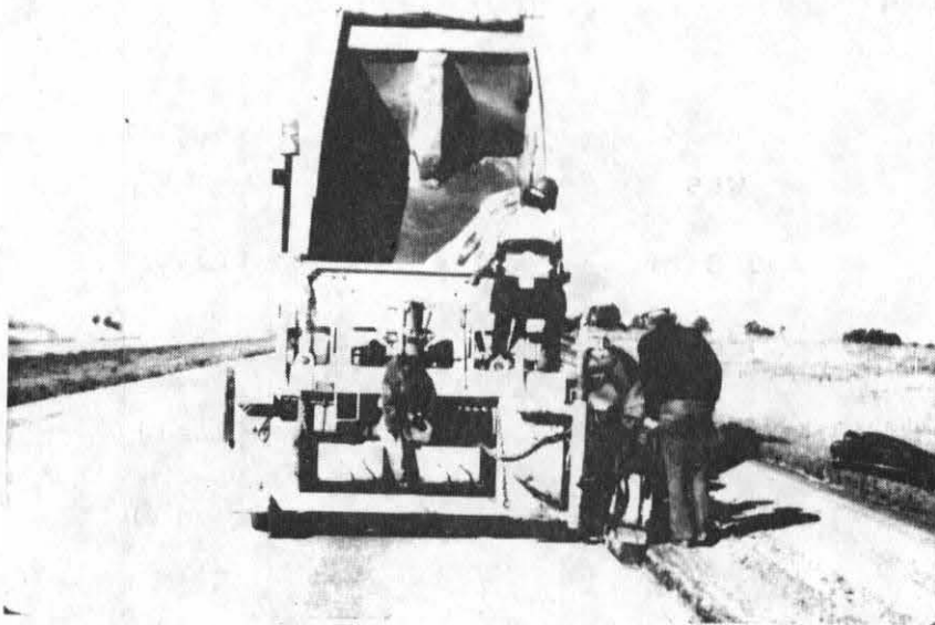
Figure 5: Blawknox RW-38 Placing Porous Backfill
