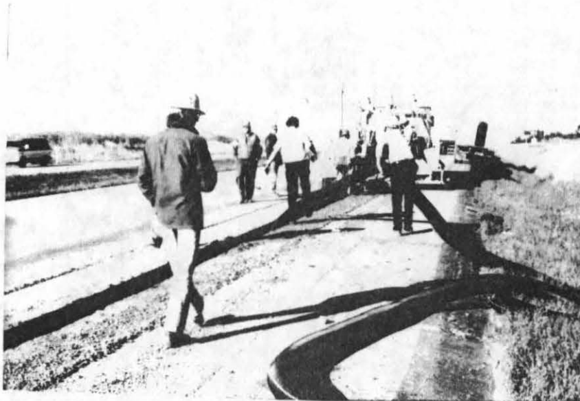
Figure 4: Hand Placement of the Tubing
