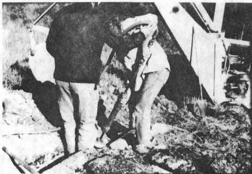
Figure 10: Tamping Earth Fill Around the RF-22 Outlets
