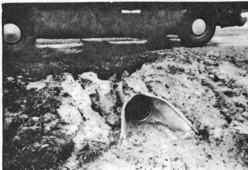
Figure 11: Erosion Around the RF-22 Outlet
