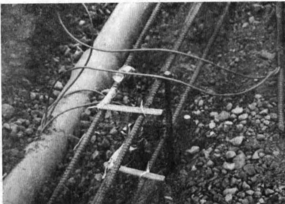
Figure 51 Installation of Concrete Gages (note: wires are only tight enough to hold gage in place)
