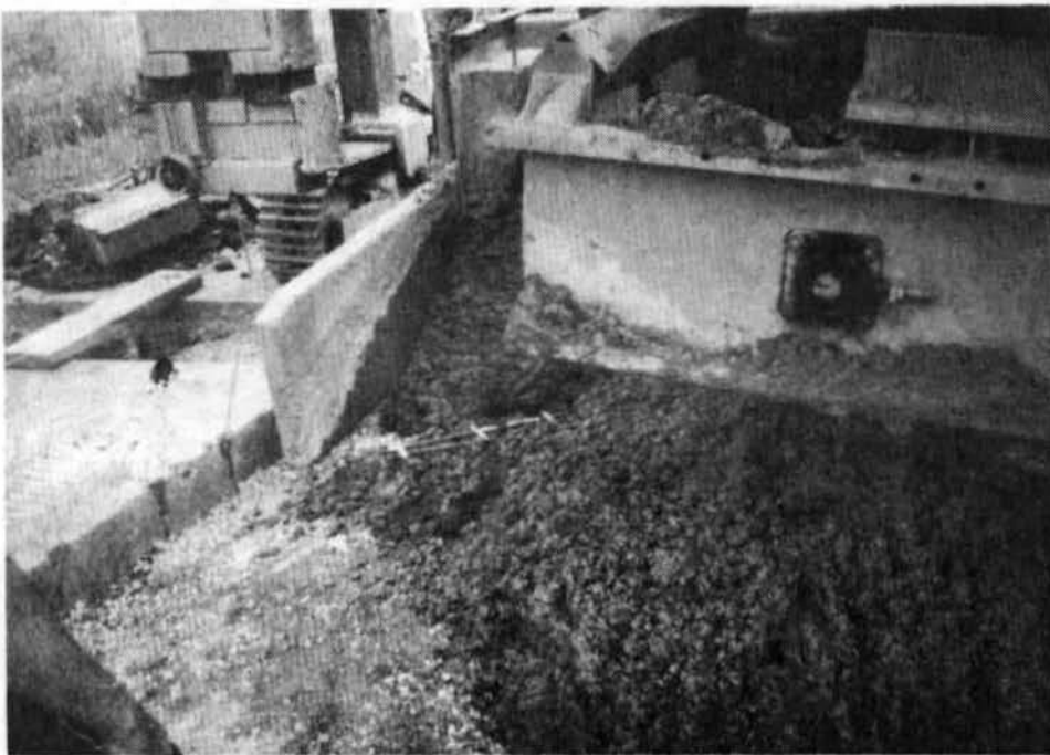
Figure 59 Concrete Placement over Corner Assemblies
