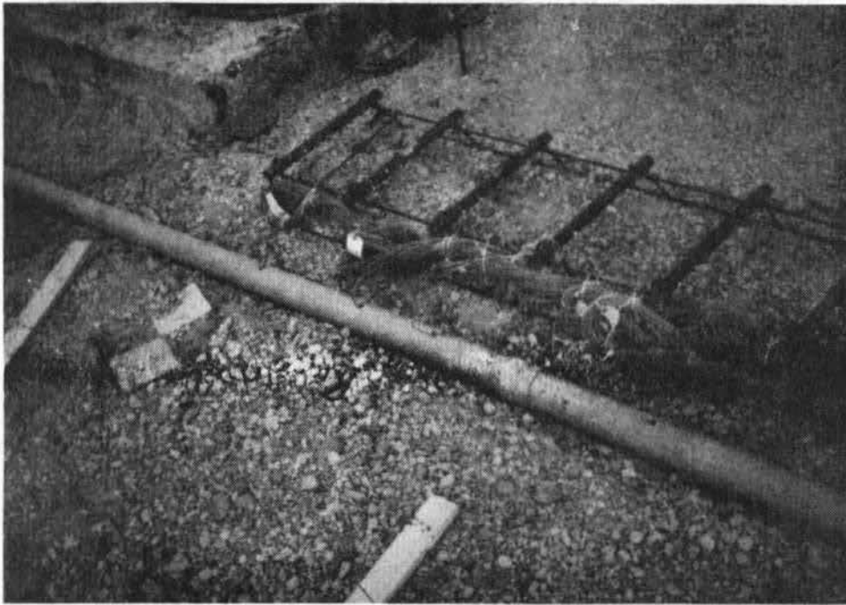
Figure 48 Dowel Bar Assembly Ready for Installation
