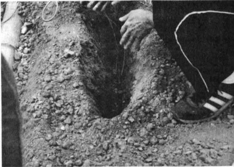
Figure 54 Installation of Temperature Gage in Base Course
