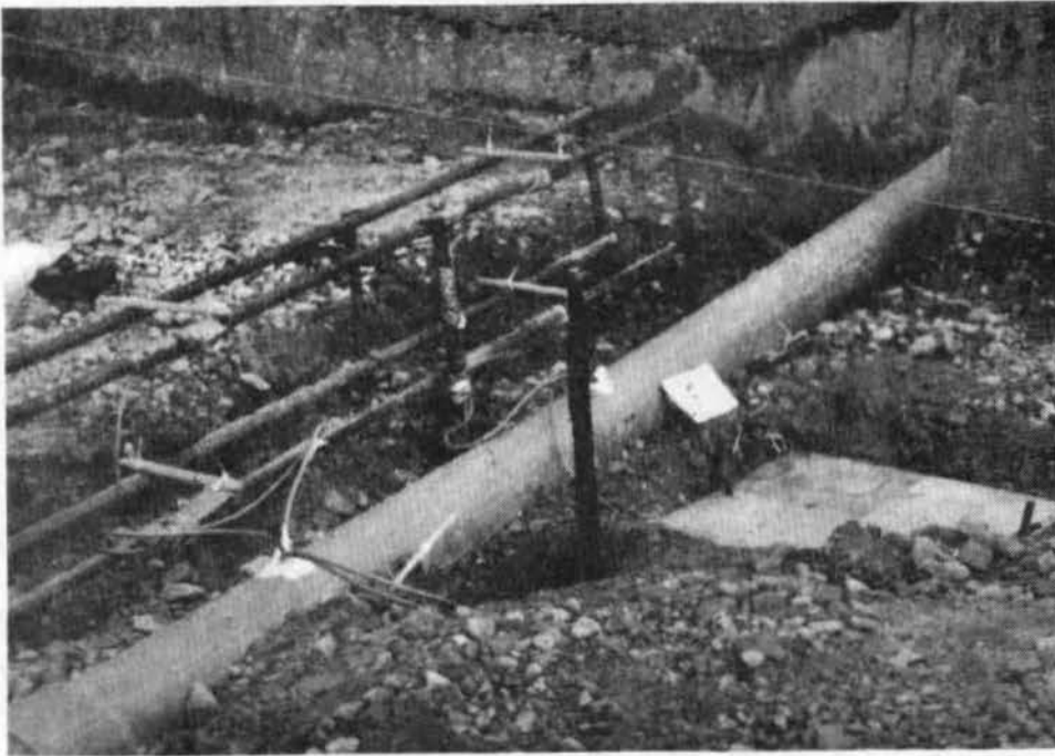
Figure 50 Placement of Carrier Conduits
