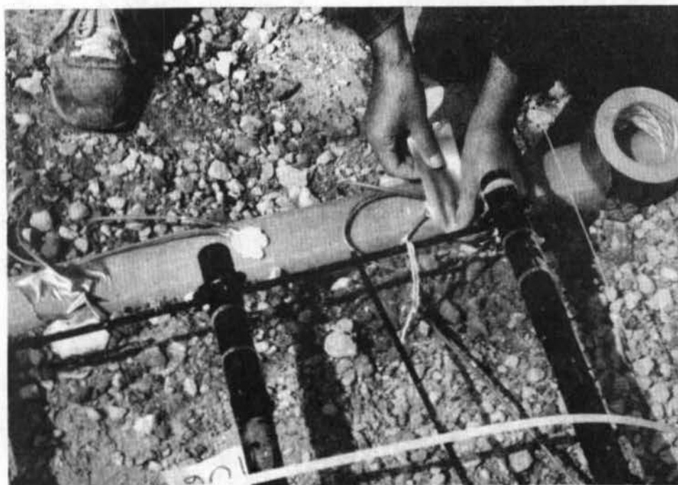
Figure 53 Completed Dowel Bar Gage Installation
