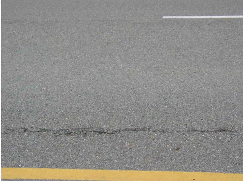
Figure A.25.3. Longitudinal crack in US 20 test section, Delaware County
