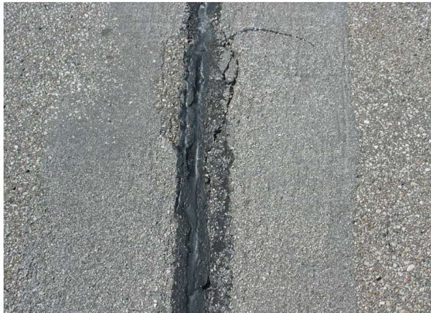
Figure A.13.4. Patching and sealed crack in G 28 test section, Muscatine County
