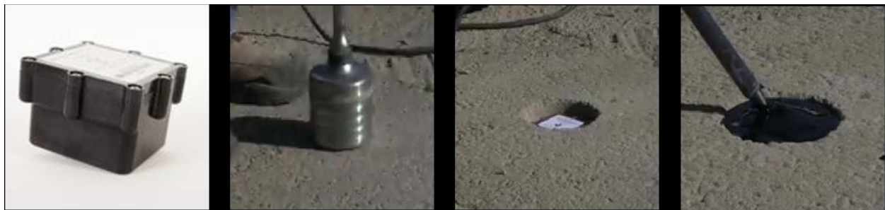
Figure 60. Wireless VDS sensor installation (Bajwa et al. 2011)
