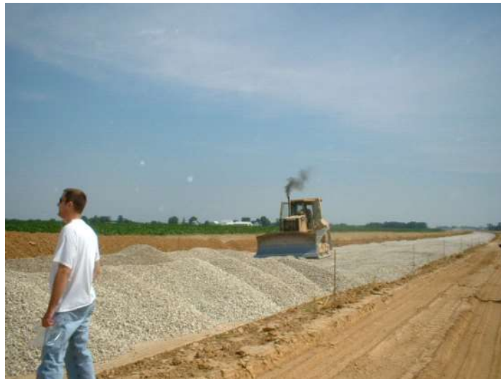
Figure 36. Spreading of aggregate piles using D6XL dozer
