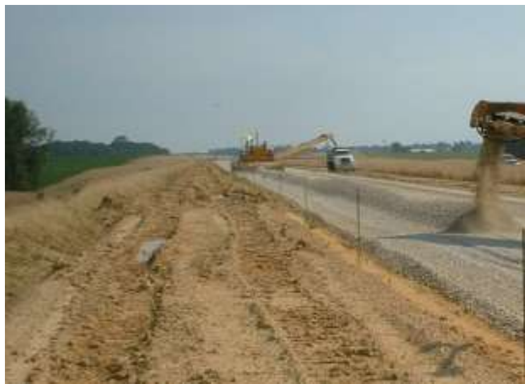
Figure 40. Placing trimmed aggregate back in to the haul trucks for re-use at other location
