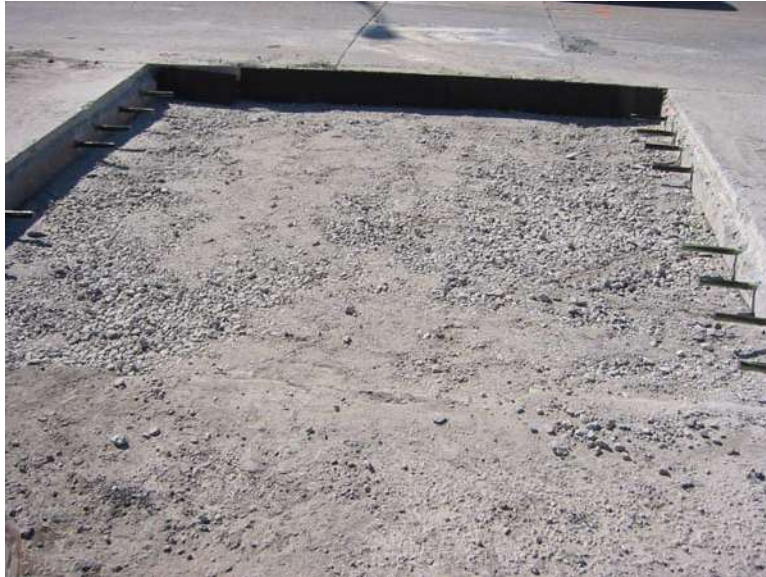
Figure 69. Recycled PCC aggregate placed over the existing subbase I-235
