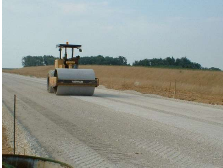
Figure 41. Final compaction using 563 CAT roller
