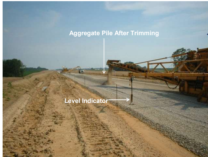
Figure 39. Final trimming of base, level indicator attached to trimmer, and aggregate pile formed after trimming
