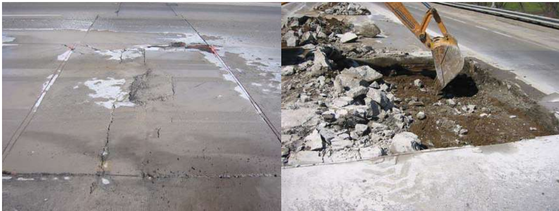
Figure 68. I-235 deteriorated PCC surface on the left, and excavation on the right
