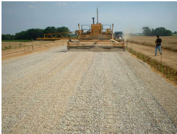
Figure 38. Final trimming using 9500 Gomanco Trimmer
