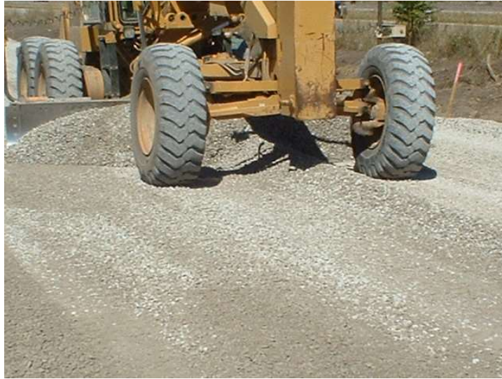
Figure 53. Spreading and trimming of aggregate
