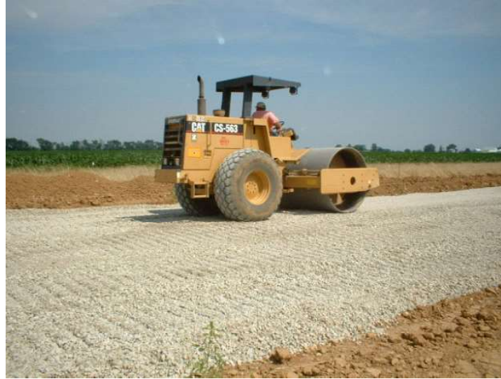
Figure 37. Initial Compaction using 563 CAT Roller
