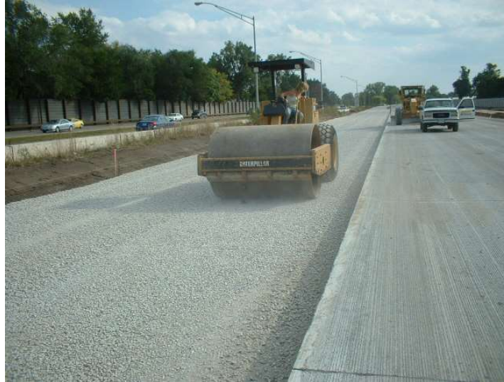
Figure 55. Roller used for final compaction
