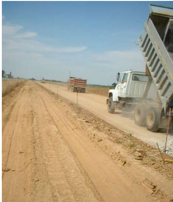
Figure 34. Unstable shoulder under loaded trucks placing aggregate
