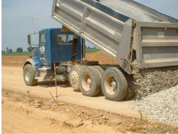
Figure 35. Dumping of aggregate on subgrade
