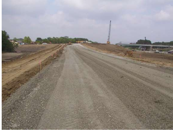
Figure 56. Photograph of the modified subbase layer during construction at 35 th street test section
