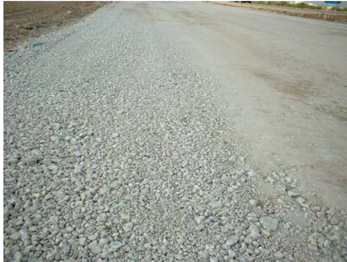
Figure 58. Picture showing segregation in fines on the final base layer
