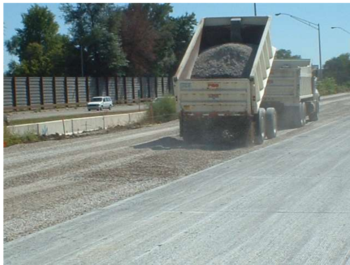
Figure 50. Dumping of aggregates from the truck
