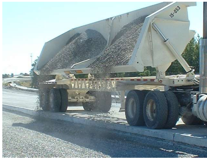
Figure 52. Another method of dumping the aggregate
