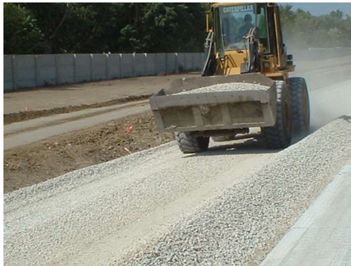
Figure 54. Bucket loader removing excess aggregate
