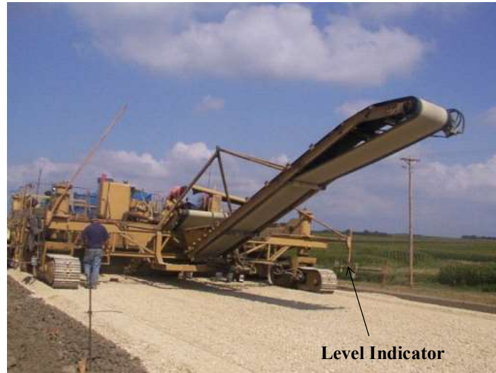
Figure 46. Final trimming process using TR 500 trimmer
