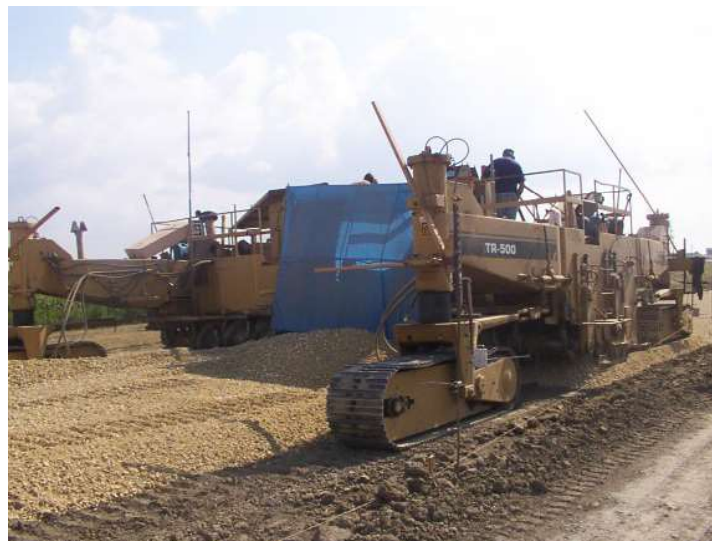
Figure 47. Piling of trimmed aggregate on the side of trimmer
