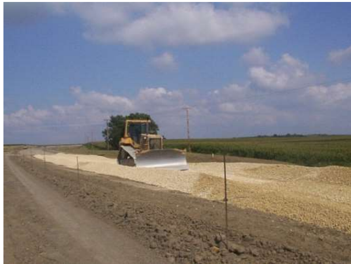
Figure 45. Spreading of aggregates using a D6XL dozer
