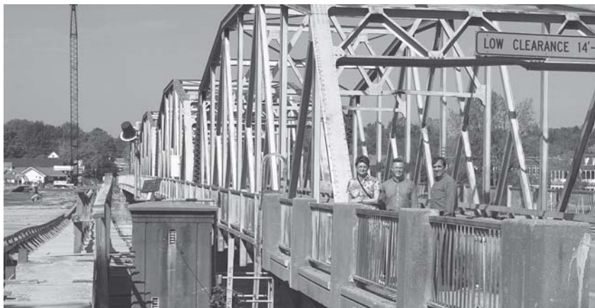
(from left) Ingrid Teboe, District 5 field services coordinator, Keosauqua Mayor Kevin Hranicka and Pete Tollenaere, assistant District 5 engineer watch construction from the old bridge.
