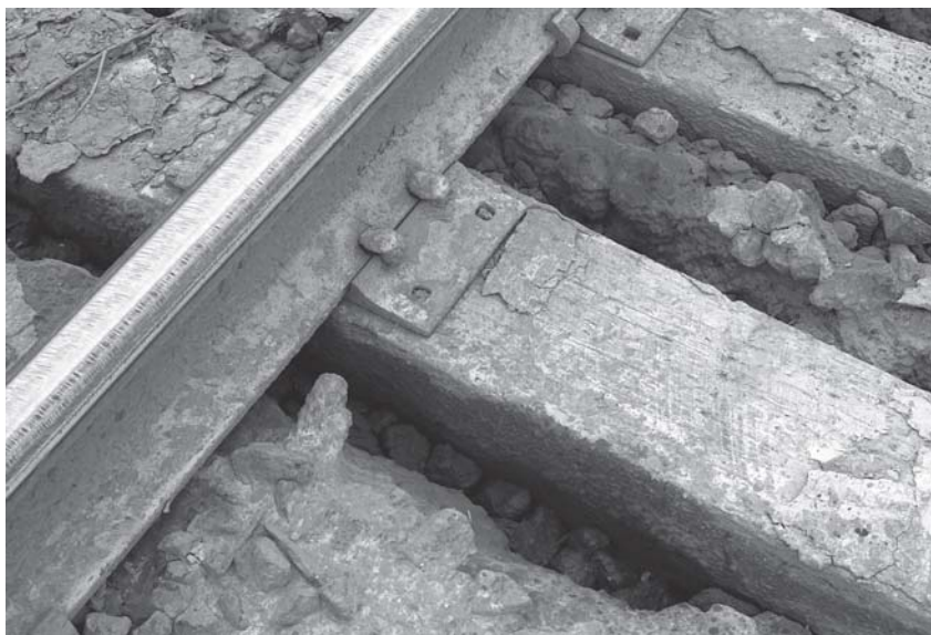
"Fouled ballast" can be a problem when the support system of a rail bed is washed away or covered in mud.
