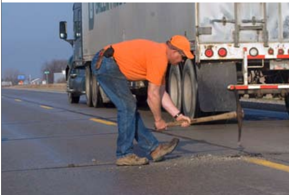
(photo left) Martin Coughenour, equipment operator in the Ames garage, removes debris from an area to be patched.
