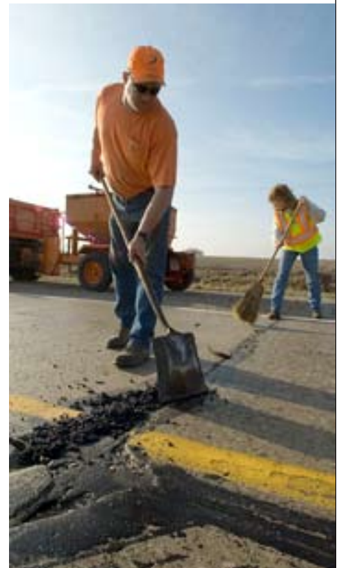
(photo left) Martin Coughenour, equipment operator in the Ames garage, removes debris from an area to be patched.
