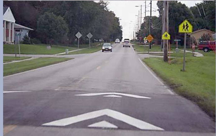
This speed table on the west entrance to Gilbert was, overall, the most effective traffic-calming technique in the study.
