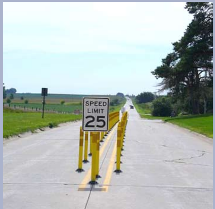
Traffic in Slater slowed considerably when these island channel markers were installed.
