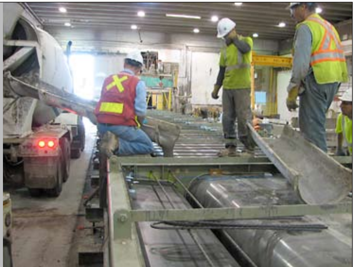
A new technology called ultra-high performance concrete is being used on some Iowa bridges. The texture of the mix is much different than traditional concrete mixes.
