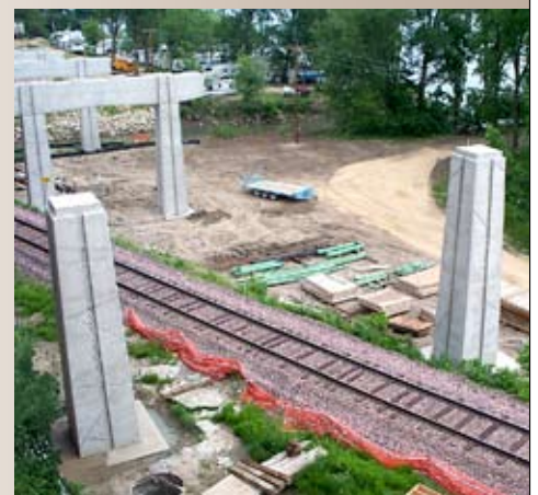
Straddle bent pier columns were used to provide adequate clearance for the railroad below the bridge
