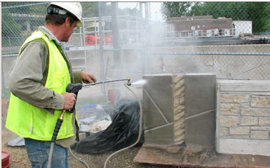
A concrete texture mock-up of a bridge tower is given a water blast finish
