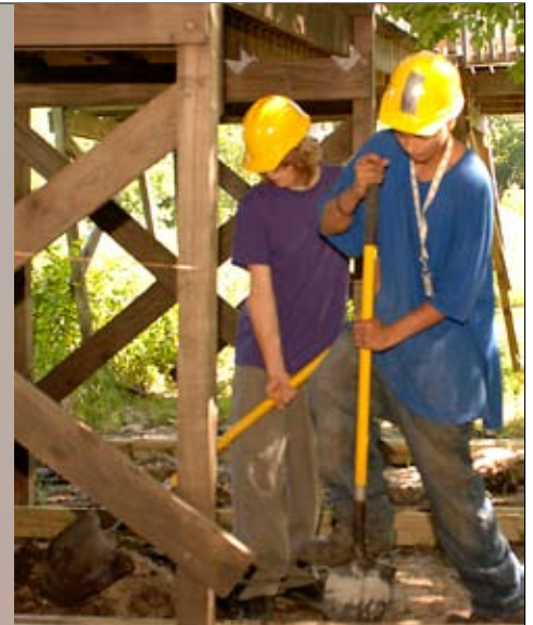
Two Black Hawk County Conservation Board UYC workers help repair a scenic overlook damaged by last year's flooding.
