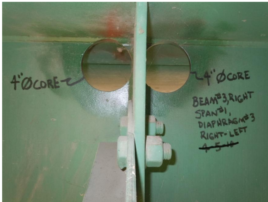
Figure 6.2.10-1. Diaphragm Connection Stiffener Fatigue Crack Retrofit
