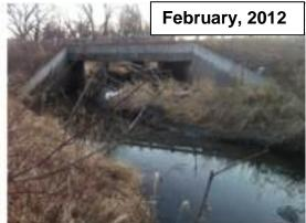
**Figure 1** Sediment deposits at a typical 3-box culvert sites in Iowa, showing the relatively fast accumulation and vegetation-stabilization of the sediment deposits
