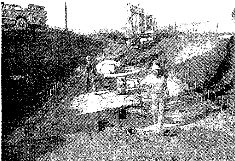
Photo 1: Metal band installation prior to balloon inflation
