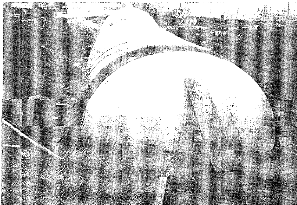
Photo 5: Concrete arch culvert in place
