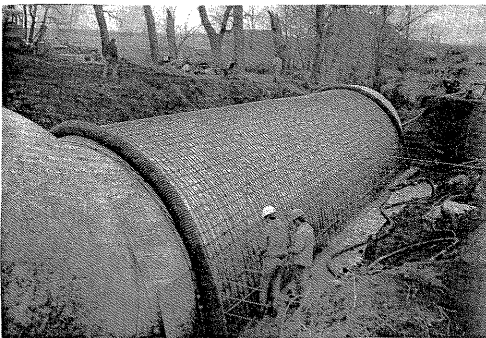
Photo 2: Reinforcing steel placement on inflated balloon
