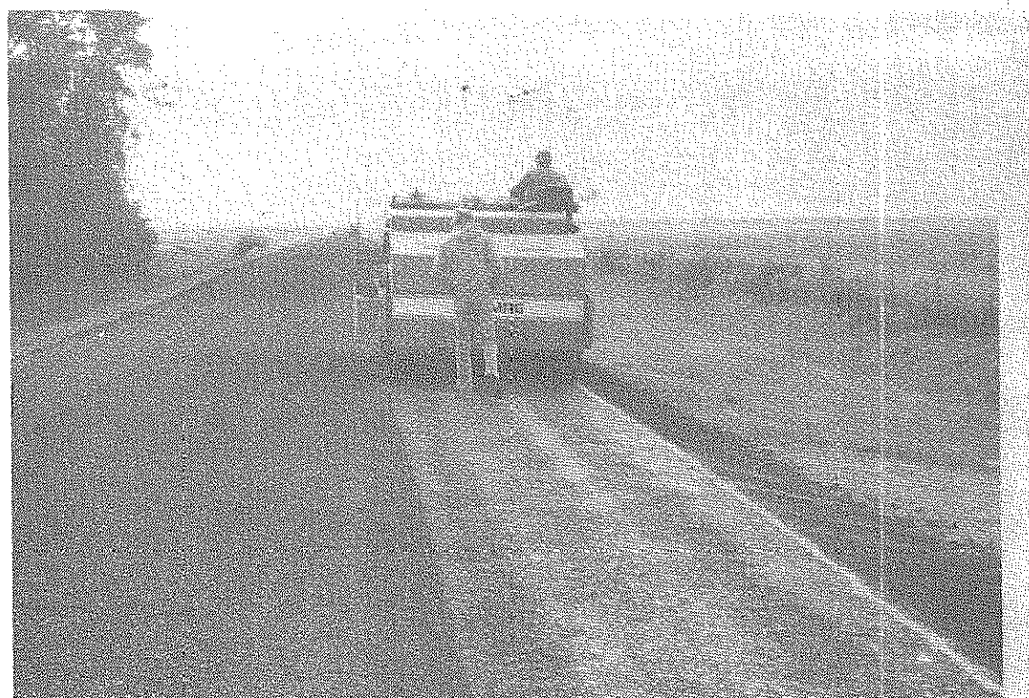
Figure 6. Compaction of road mix section
