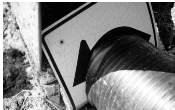
Figure 37 An old road sign was used to protect the end of the liner during insertion. Note that there is still some deformation.
