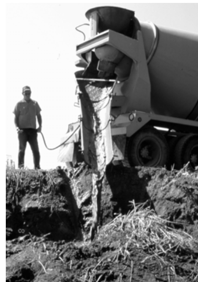
Figure 18 Mortar was delivered and placed with an ordinary ready-mix truck.
