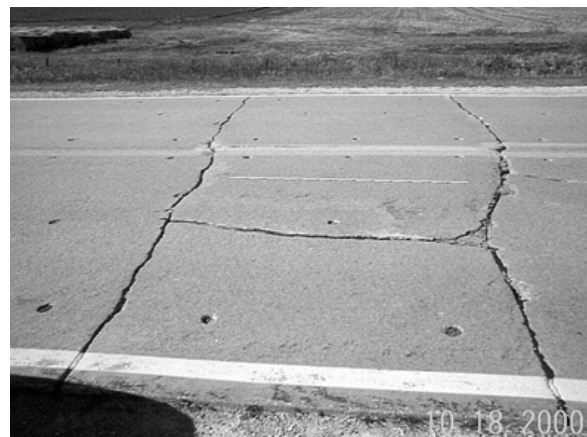
Figure 65 Pavement over culvert showing settlement cracking and mud-jacking holes.
