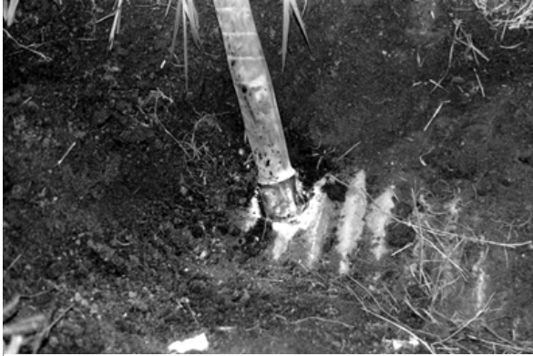
Figure 7 Pumping grout into annulus through access.
