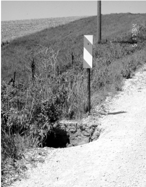
Figure 11 Section of roadway that was subsiding into the old culvert.
