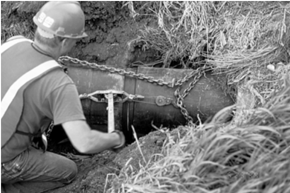
Figure 50 Joining the first and second segments.
