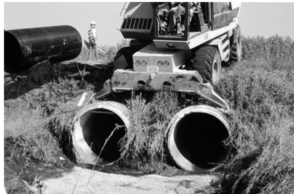
Figure 23 Original culverts with back hoe in place to assist with liner insertion. Note the aggregate placed to try to stabilize the soggy ground.
