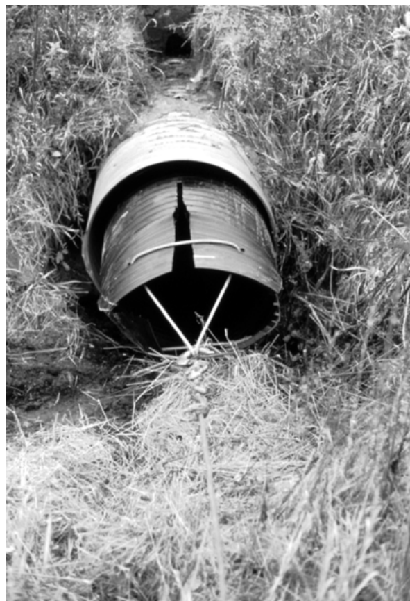
Figure 44 Pulling the liner through the culvert.
