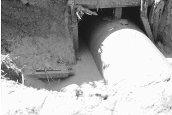
Figure 19 Mortar is half-placed. Note brace above the liner.
