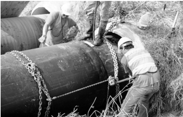
Figure 29 Connecting two Snap-Tite™ liner segments together using chains and winch.
