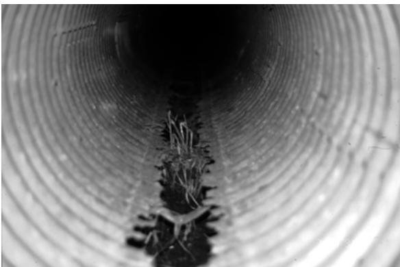
Figure 33 Bottom of original culvert.
