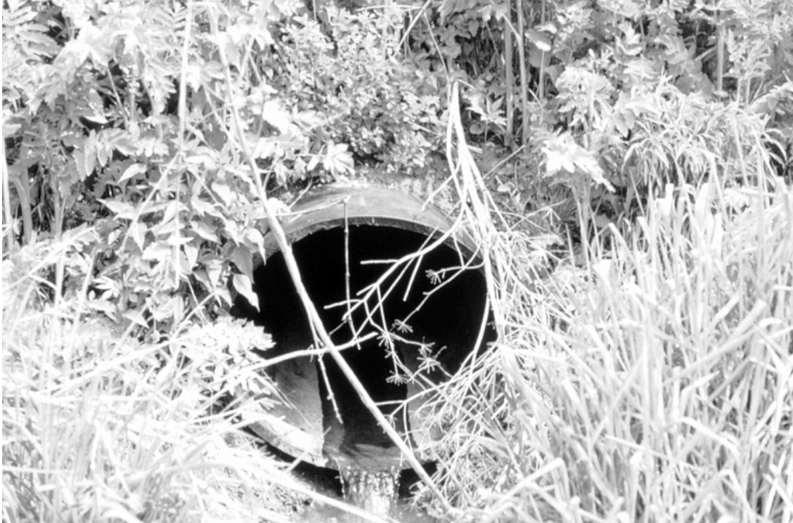
Figure 22 View of the south end of the culvert as it appeared in 2001.
