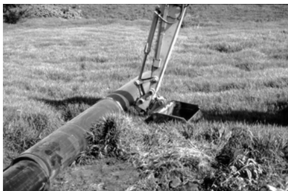
Figure 12 Unloading and aligning the two segments.
