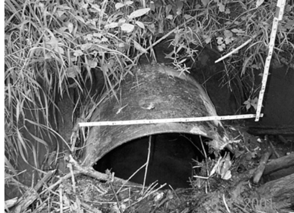
Figure 85 The inlet to the lined culvert, also at about six years. It was mostly covered and clogged with debris (some of which was removed for this photograph).
