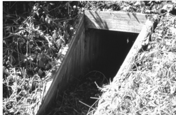
Figure 9 North end of original culvert.
