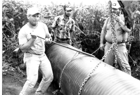
Figure 3 Threading two liner segments together.
