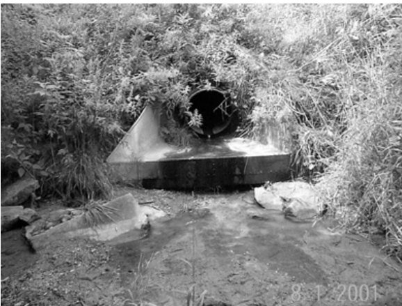
Figure 84 This is the outlet of the lined culvert after about six years. The headwall for this end was constructed from metal instead of concrete.
