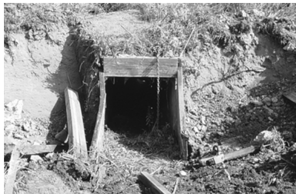
Figure 13 North end after clearing.
