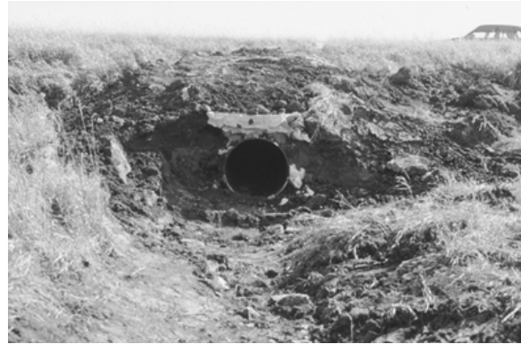
Figure 66 Grouted "headwall" at the downstream side of the lined culvert.
