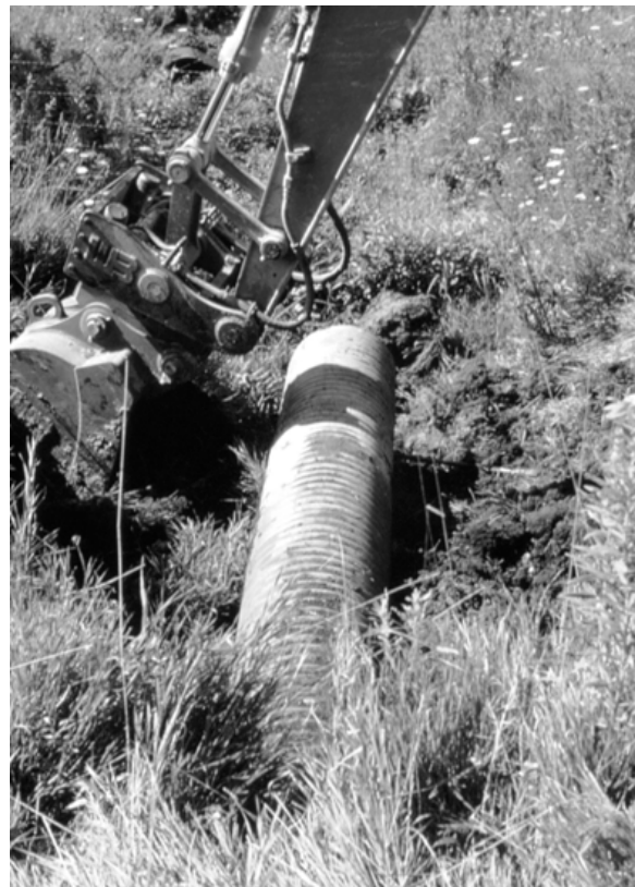
Figure 34 Clearing around the existing culvert to enable adjustment of the alignment.
