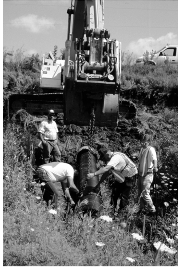
Figure 35 Placement of the first liner segment.
