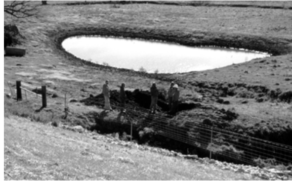
Figure 42 Clearing of work area at south end of culvert.
