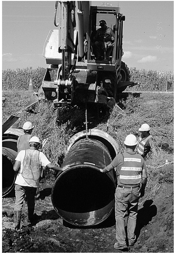
Figure 30 Inserting the Snap-Tite™ liner into the east culvert.
