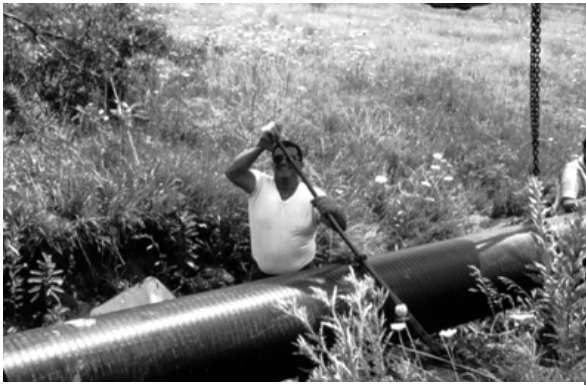
Figure 36 Threading two liner segments together.
