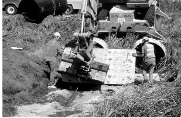
Figure 28 Inserting the Culvert-Renew™ liner into the west culvert with a piece of plywood to protect the end of the liner from the back hoe bucket.
