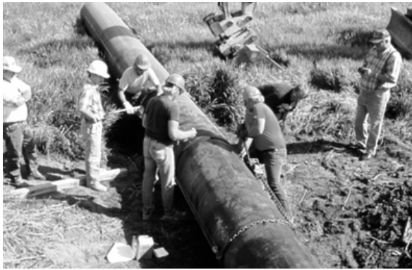
Figure 15 Coupling of liner segments.
