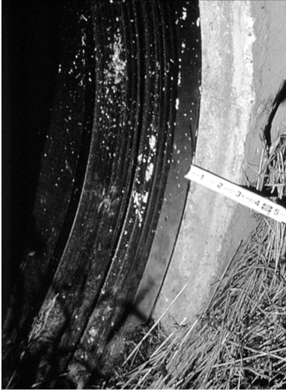
Figure 58 Movement of the liner with respect to the headwall on the north side.
