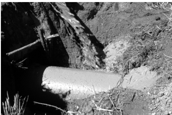
Figure 17 Mortar being poured into annulus in front of earthen dam.
