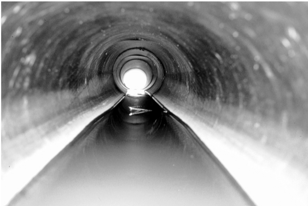
Figure 21 View of the inside of the lined culvert several years after construction. Note the indentations in the top of the liner from the grouting pressure.
