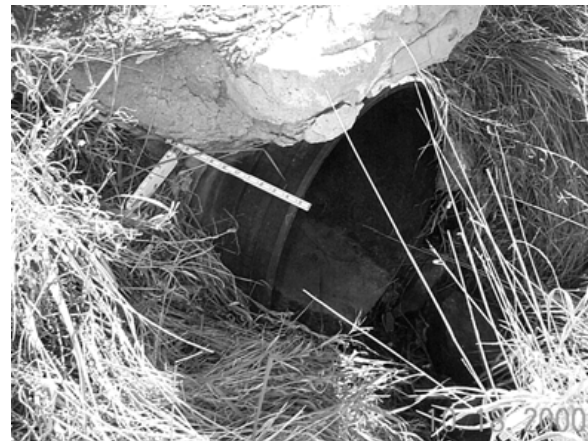
Figure 68 Grout covering on the downstream side after several years of erosion of the slope around it. This piece subsequently broke off and rests in the ditch below.
