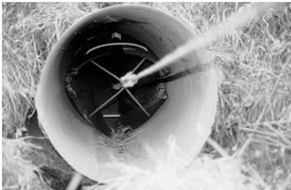
Figure 43 Cable attached to the cone at the front of the liner.
