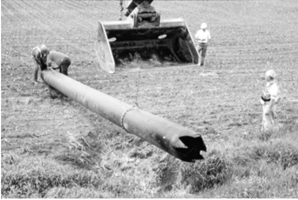
Figure 48 Maneuvering the first liner segment into position.
