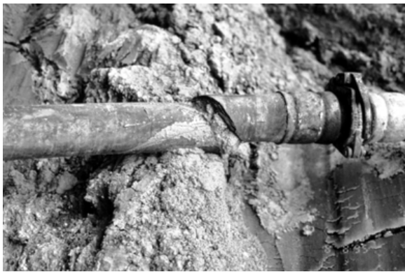
Figure 82 This is what happens if the pumping is stopped to wait for a second ready-mix truck.
