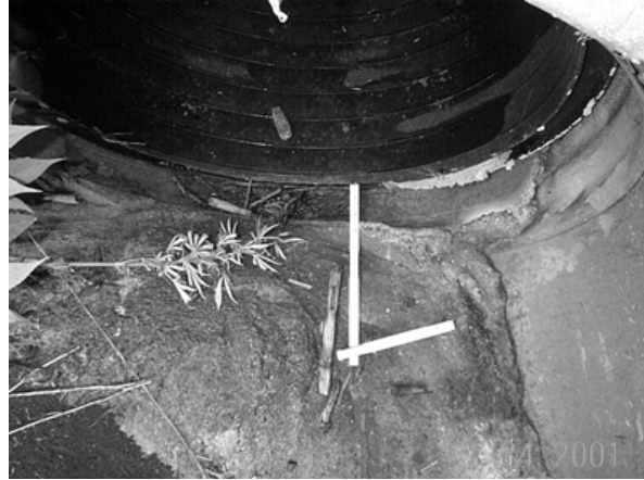
Figure 8 Close-up of north end showing liner movement.
