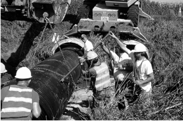
Figure 27 Connecting two Culvert-Renew™ liner segments together using a strap wrench.
