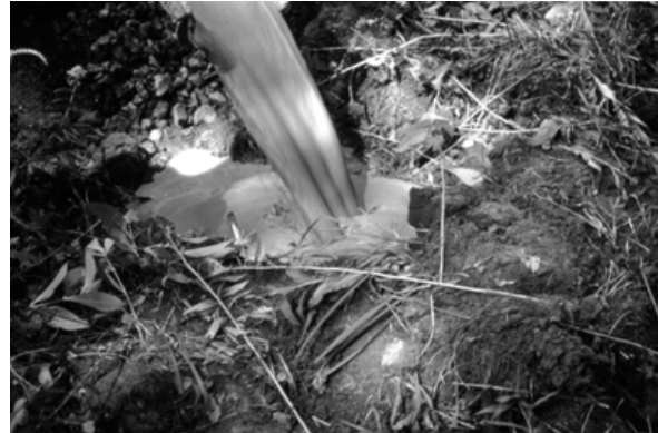
Figure 62 Pouring the grout.
