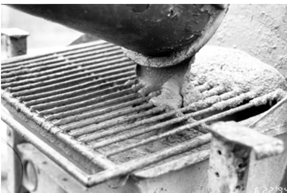
Figure 6 Pouring grout into concrete pump hopper.
