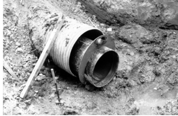
Figure 83 After the problem shown in the last photograph, it was impossible to pump more grout into the outlet end. The remaining mortar was pumped into the inlet end of the lined culvert.
