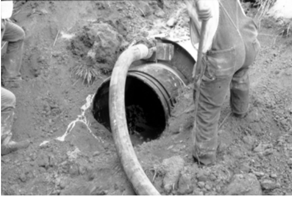
Figure 80 Pumping grout into the annulus at the outlet end.
