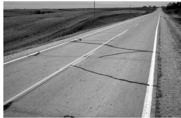
Figure 60 Cracking that appeared above the culvert. These cracks were not observed in the previous inspection (2001).
