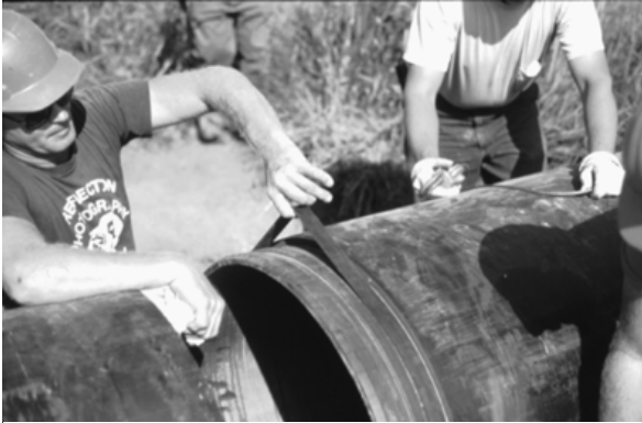
Figure 14 Joint between two segments showing sealing strap.
