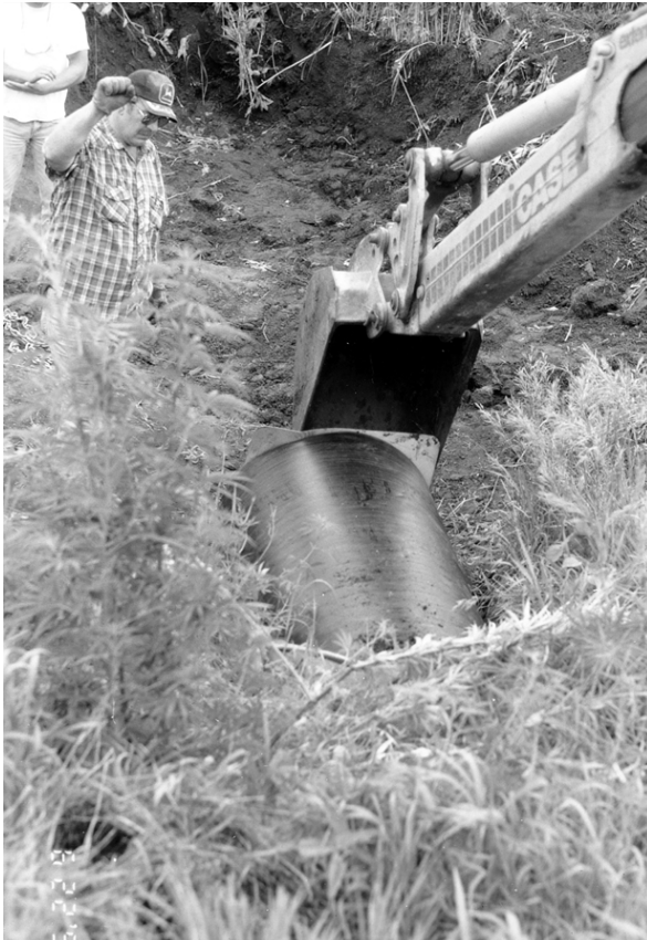
Figure 4 Inserting liner section into culvert with a backhoe.
