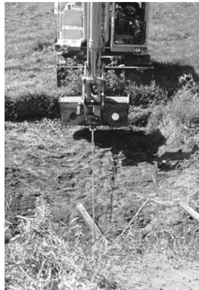
Figure 16 Pulling the liner through the culvert.
