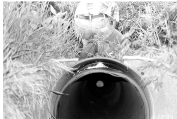
Figure 5 Cutting grout access holes in original culvert.
