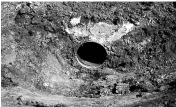
Figure 67 Grout at upstream side of lined culvert.
