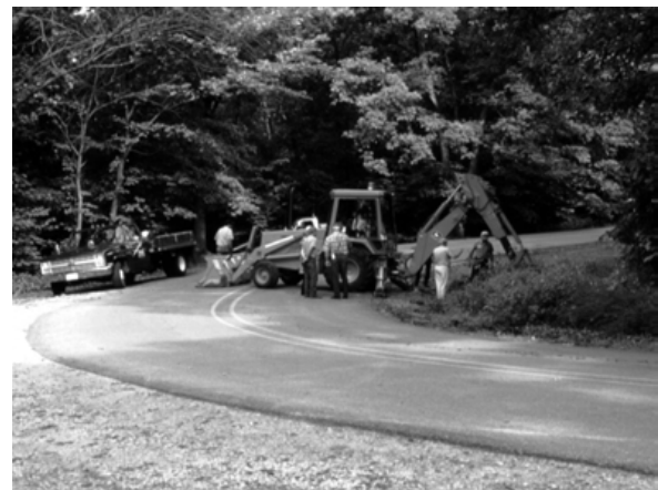
Figure 61 Equipment in place to insert the liner.
