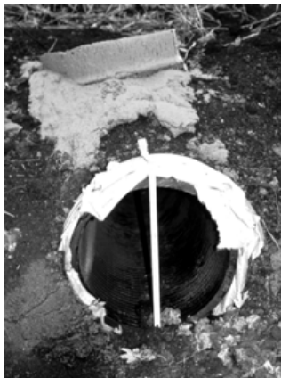
Figure 69 Inlet end of lined culvert. The annulus was blocked for grouting with fiberglass fabric. Note the funnel above the liner. It was the same design as the first Mahaska project.
