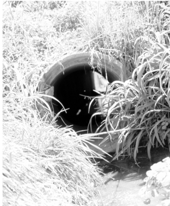
Figure 10 South end of original culvert with a short segment of PCC pipe inserted.
