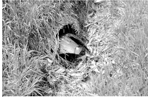
Figure 51 Appearance of "bullet nose" at the other end of the culvert.
