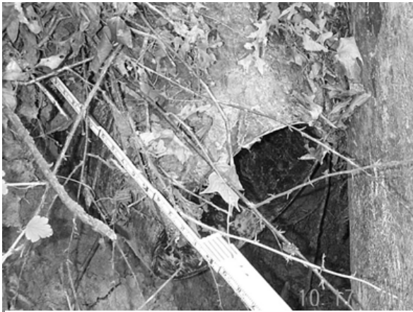
Figure 63 West end of lined culvert after about six years.
