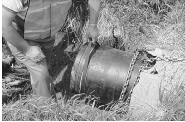
Figure 49 Preparing joint for adding the second segment.
