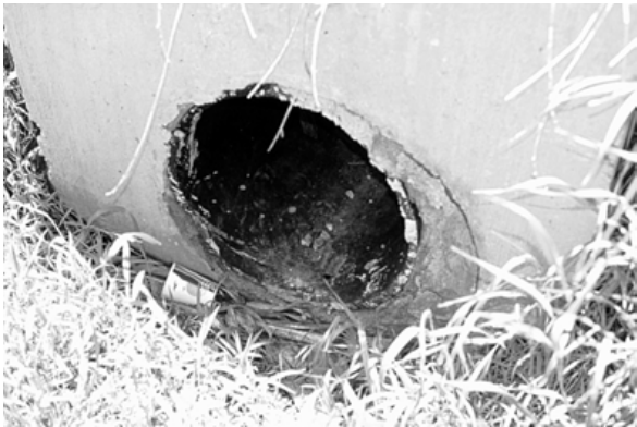
Figure 52 Headwall for the east culvert.
