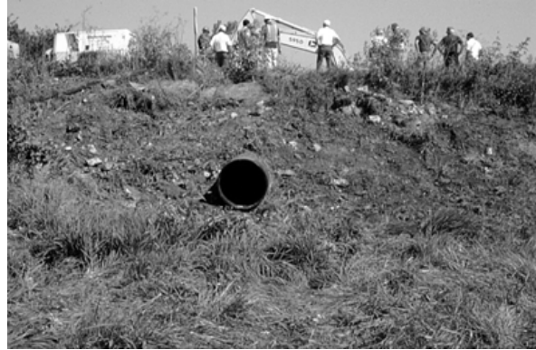
Figure 20 South side of culvert after slip-lining was complete.
