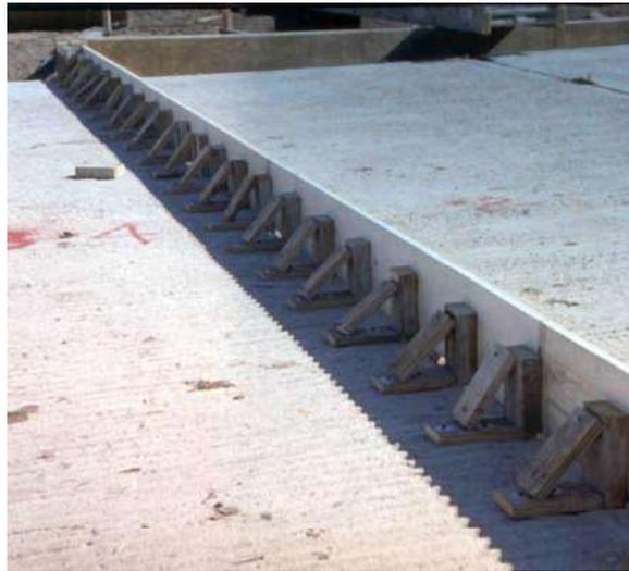
Figure 3.19. Formwork at bridge centerline for CIP deck placement.
