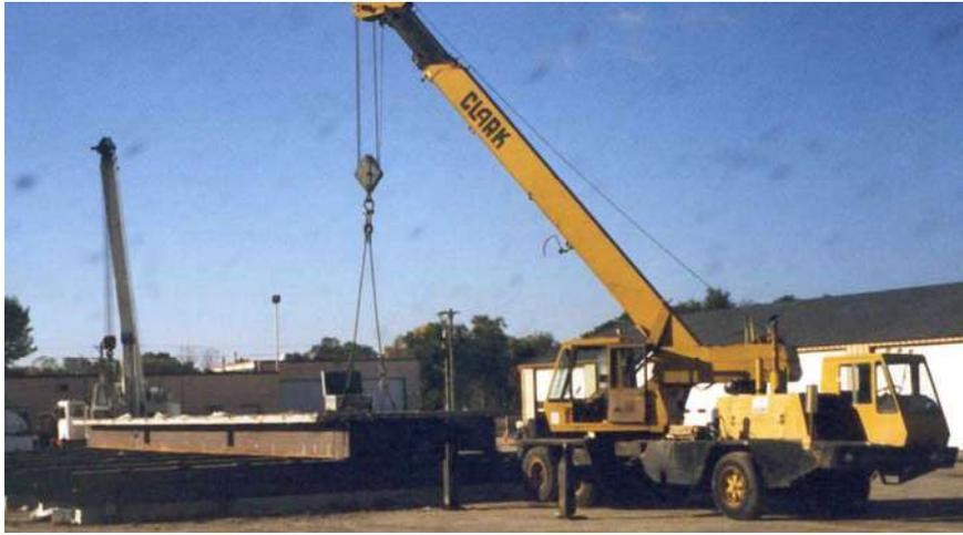
Figure 3.16. Photograph of lifting one PCDT unit at county maintenance facility.
