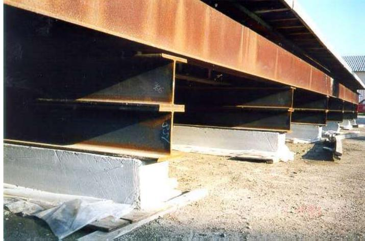
Figure 3.9. Photograph of the temporary supports used during fabrication of PCDT units.
