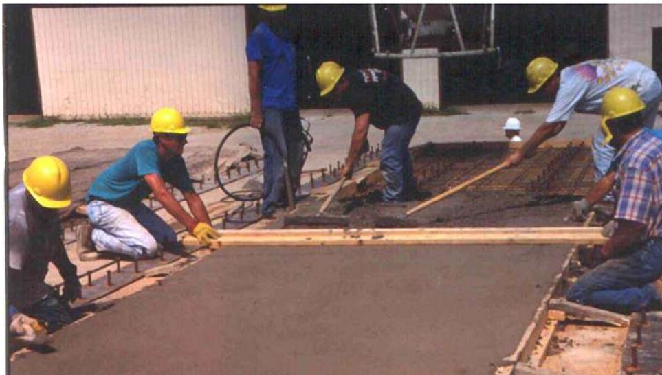
Figure 3.14. Concrete placement operation for PCDT units.
