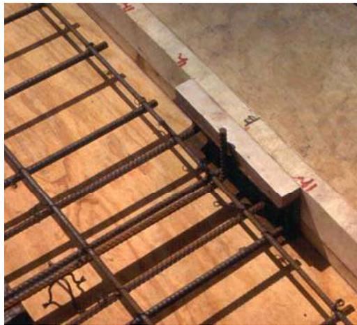
Figure 3.13. Wood blockout covering PC connector.
