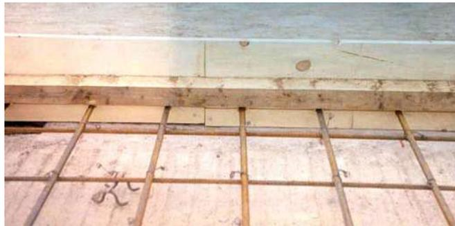
Figure 3.20. Photograph of the keyway placed on longitudinal formwork.
