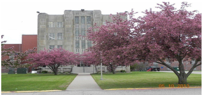
Mt Pleasant Correctional Facility
