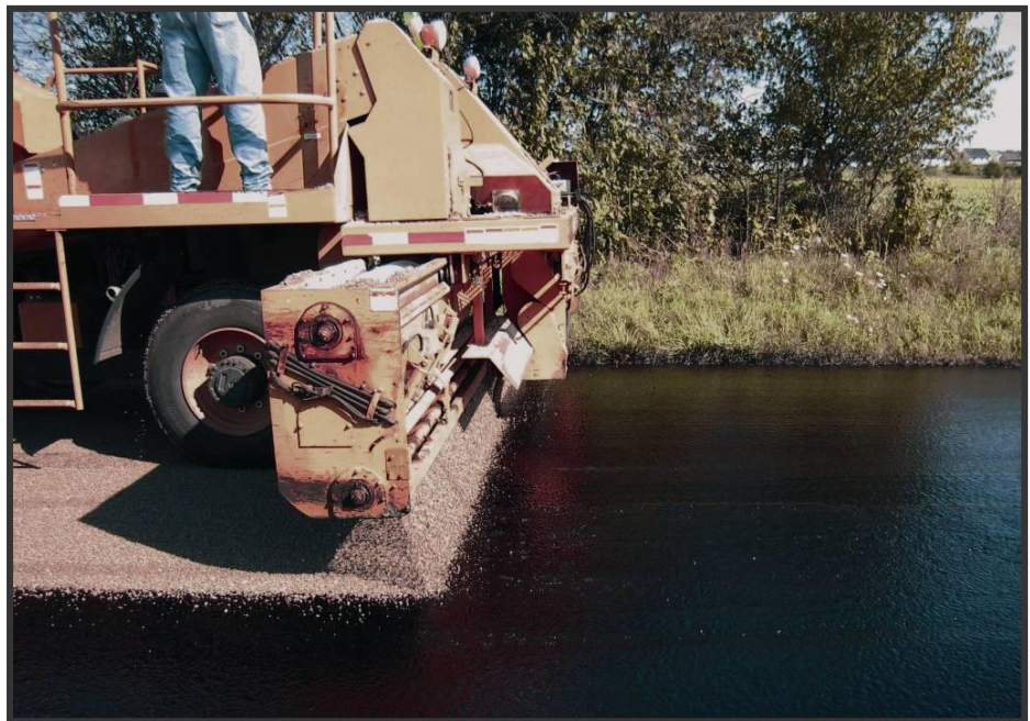
A chip spreader applies cover aggregate during a seal coat or "chip seal" operation on 74 th Street in Cedar Rapids, Iowa, during a road maintenance effort
