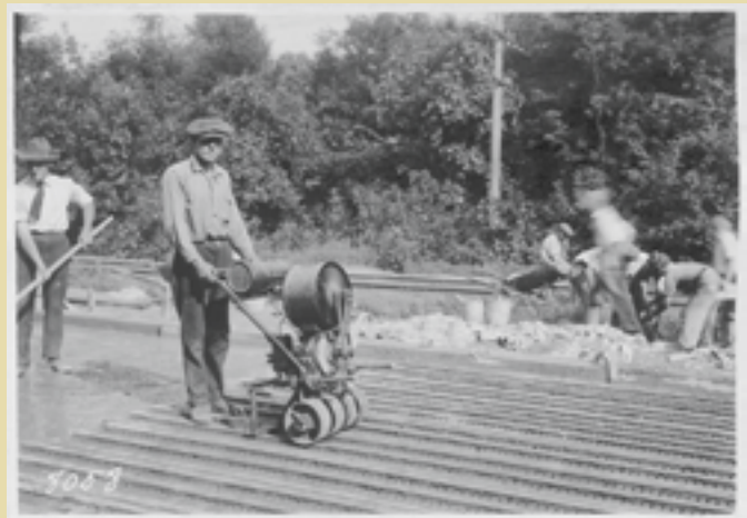
Man using a paving machine in Black Hawk County, circa 1921
