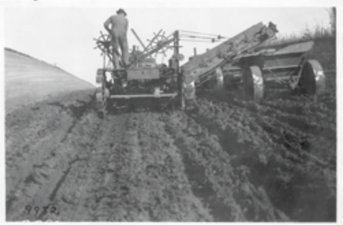
Shirley motorized grading equipment being used in Crawford County, circa 1922
