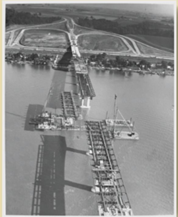
Aerial view of center span of Le Claire bridge to carry Interstate 80 over the Mississippi River, circa 1966. The bridge is being repaired this construction season.
