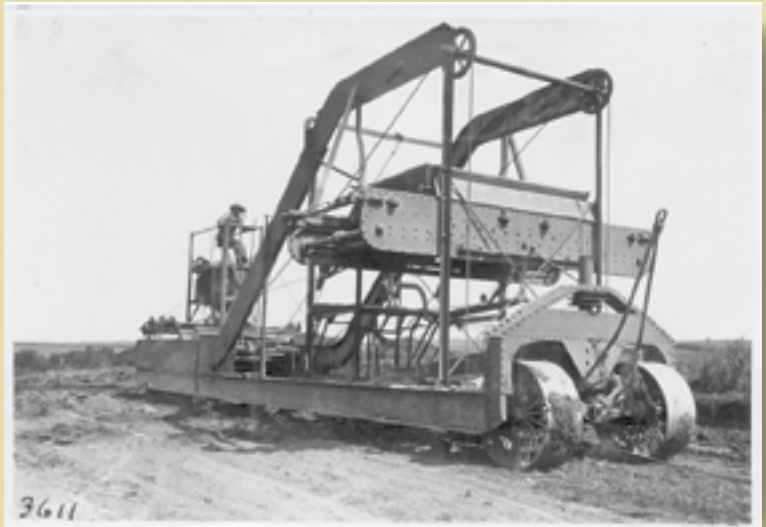
Road building equipment used by contractor L.C. Wood in Hardin County, circa 1916
