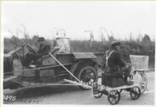
Men painting white center strip on paved road in Black Hawk County, circa 1923 (note "the slow poke" sign on the painting wagon)
