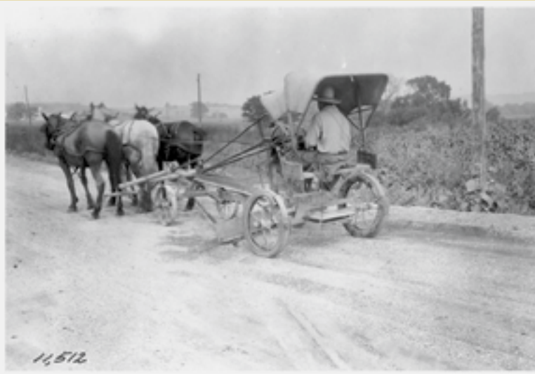
Horse-drawn covered grader on highway 13 and 18 at McGregor, circa 1926
