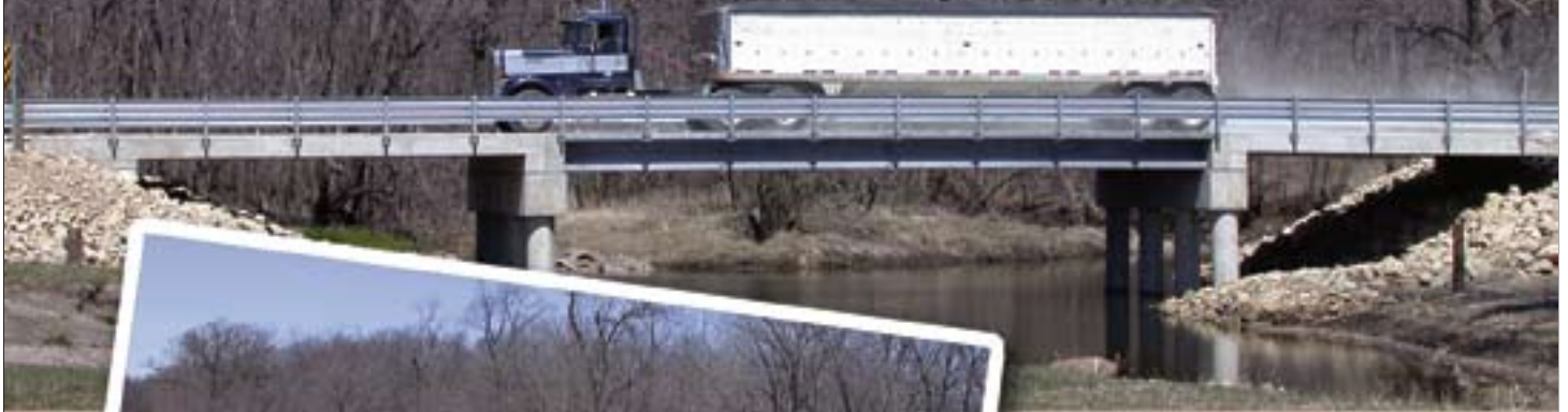
(top) Buchanan County is home to the first North American highway bridge built with the latest technology in ultra-high performance concrete (UHPC). The new Jakway Park Bridge replaced a structure built in 1910.
