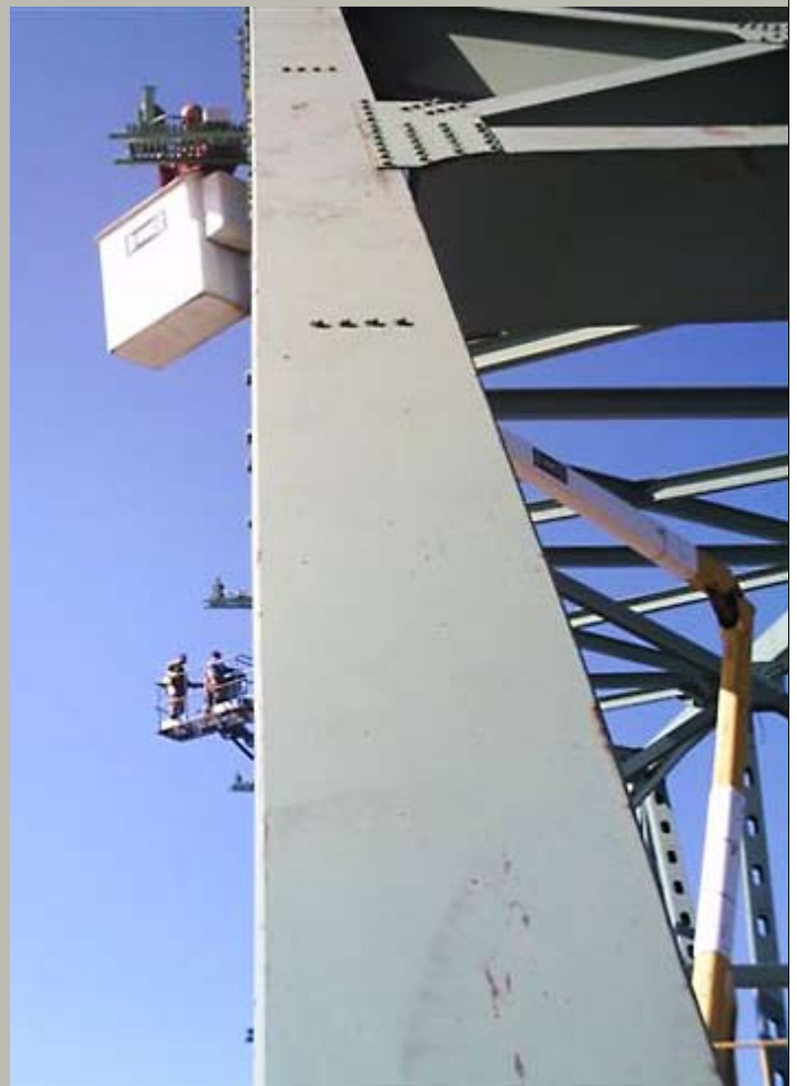
Workers from Nelson Electric install lighting on the Muscatine Bridge.
