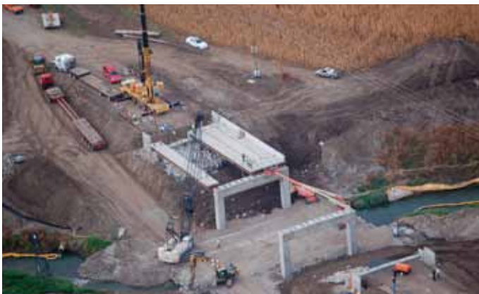
Two large cranes lift the precast bridge deck into place.
