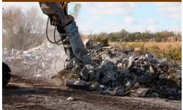
The old U.S. 6 bridge was crushed and the concrete rubble used as rip rap.
