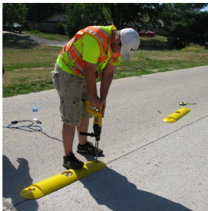
Installation of raised curbing using bolts
