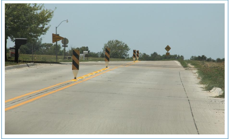
Mountable curbing installed at west St. Charles community entrance
