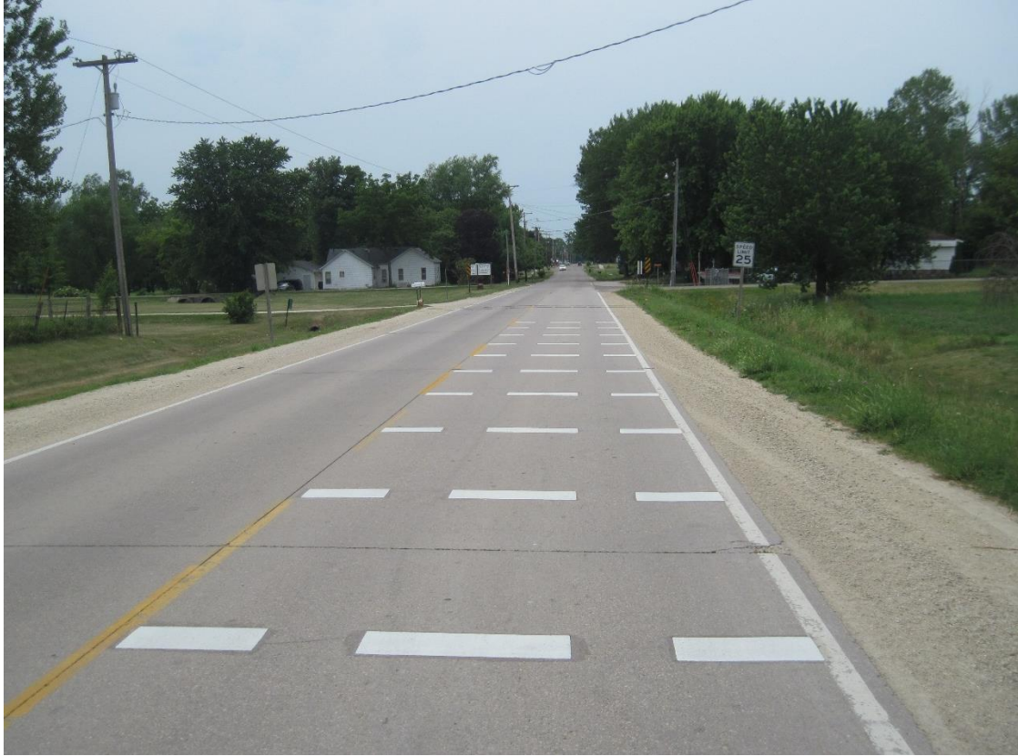
Figure 5-2: Transverse bar treatment at Hazleton east entrance
