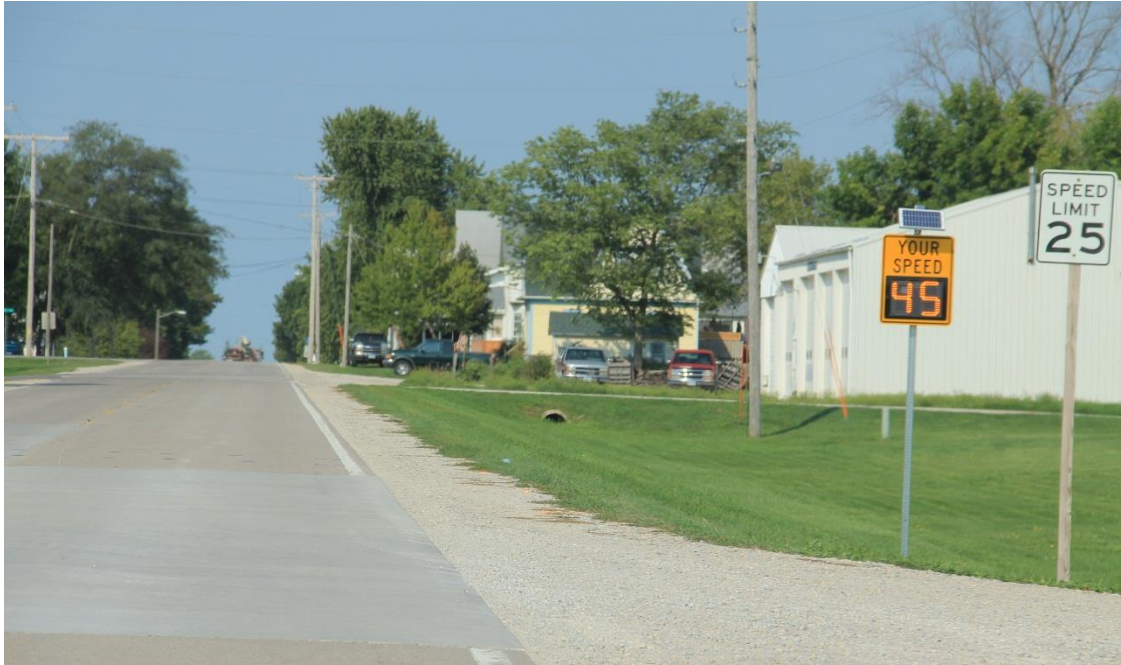
Figure 5-17: DSFS installed at east Rowley community entrance
