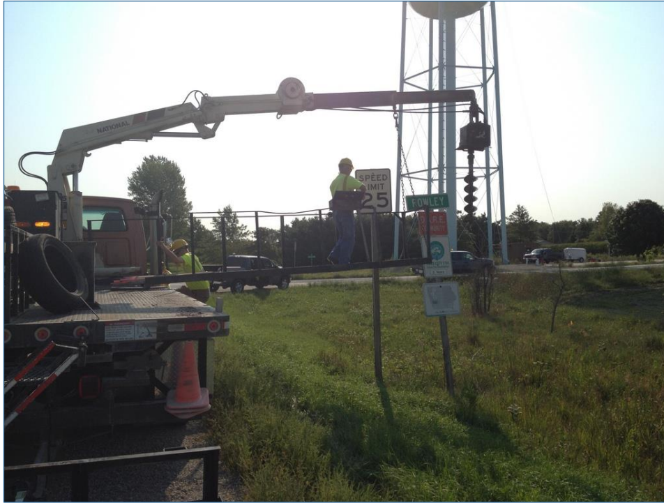
Figure 3-13: Installation of LED speed limit sign
