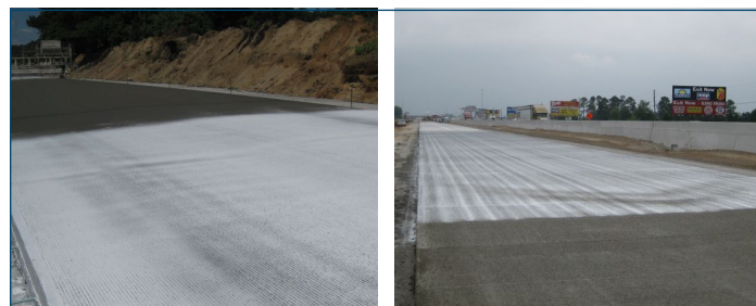
Figure 58. Poor curing practice
