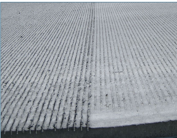
Figure 18. Nonuniform texture depth across width of transverse tining rake
