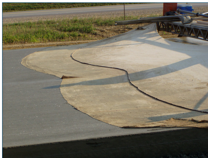
Figure 54. Burlap drag attached to a work bridge
