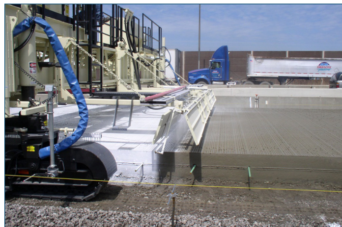
Figure 57. Illustration of curing equipment on texture-cure machine following good practice
