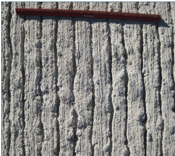
Figure 15. Excessive intermediate aggregates in close proximity to the surface leading to undesirable texture
