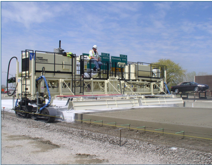
Figure 48. Texture-cure machine manufactured by Guntert & Zimmerman
