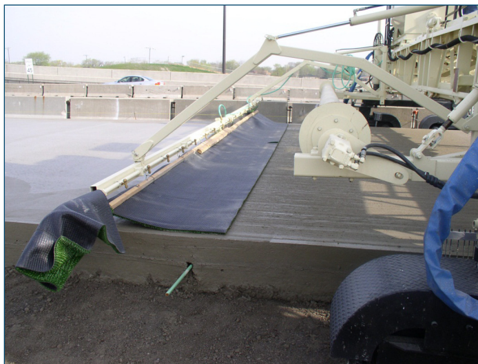
Figure 53. Turf drag attachment on a texture machine
