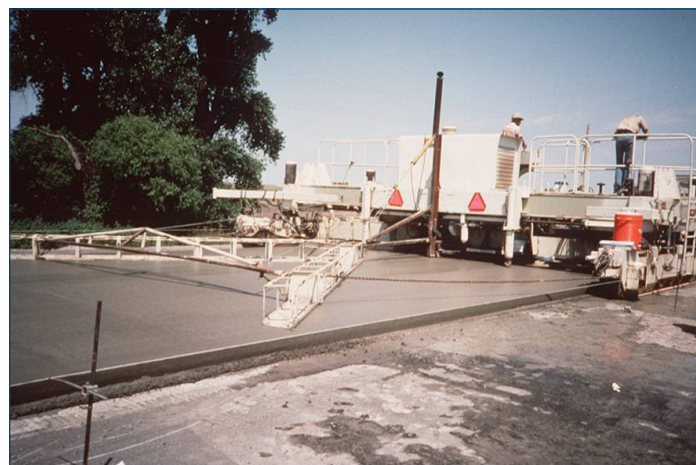
Figure 45. An alternative chevron-type float attachment for a paver
