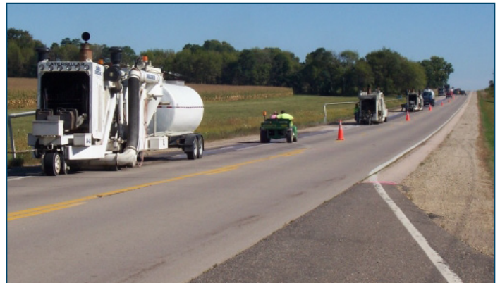
Figure 59. A grinding large-scale concrete pavement resurfacing operation
