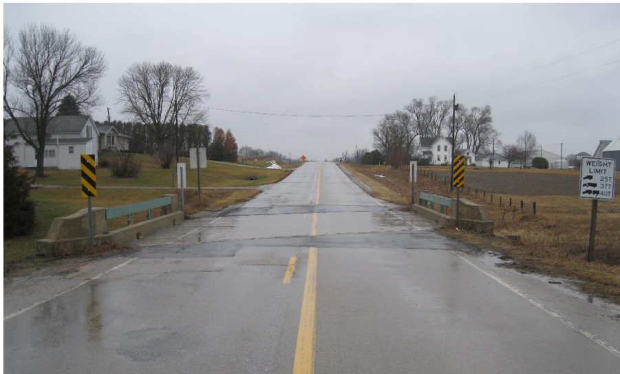
Figure 2. Johnson County Bridge end view
