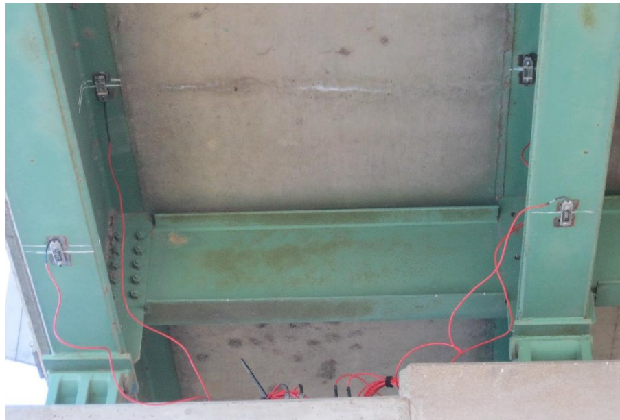
Figure 10. Sioux County Bridge instrumentation setup
