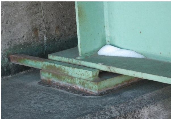
a. Abutment bearing
