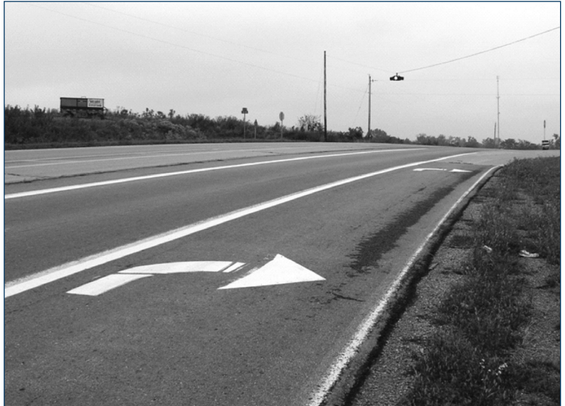
Offset right-turn lane looking northeast along IA-137. (Courtesy of Ryan Pettit, ISU)
