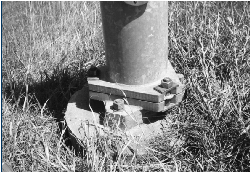
Close-up of a breakaway base on a lighting pole. (Courtesy of the Iowa DOT)
