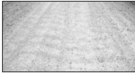
If corrugations like these aren't repaired, they'll turn into . . .
