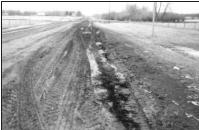
Water ponding on the shoulder (above) indicates inadequate roadside drainage.
