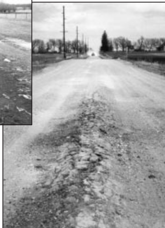
Water ponding on the shoulder (above) indicates inadequate roadside drainage.
