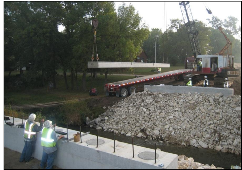
b. Unloading of Beam #4
