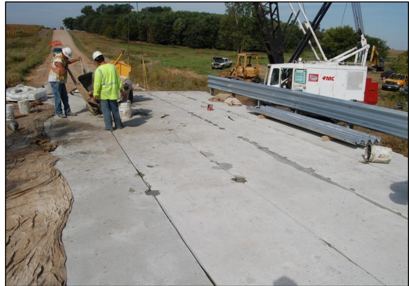
l. Placement of non-shrink grout
