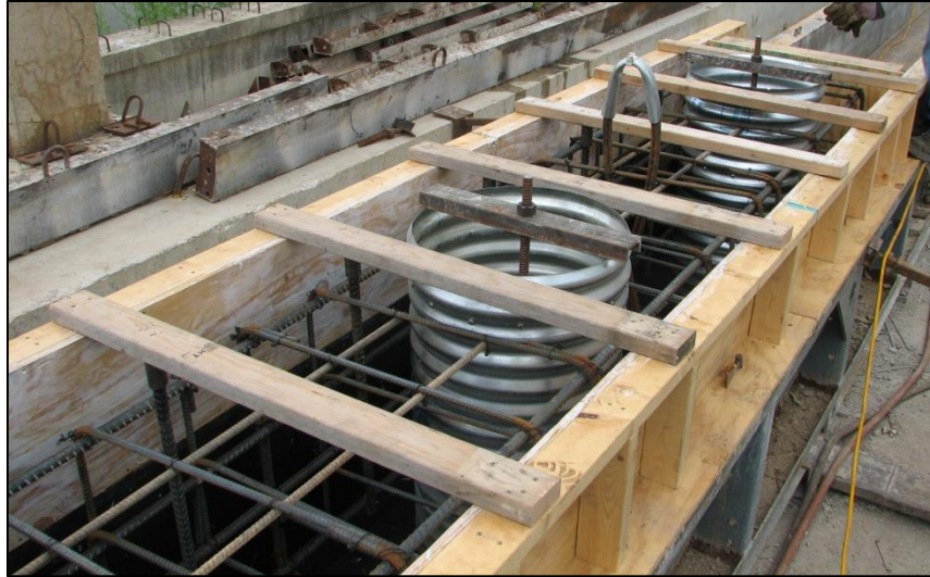
Figure 2.12. Abutment cap forms
