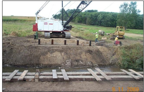
d. Piling completed in west abutment
