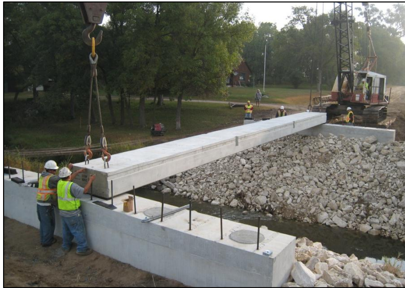
c. Positioning of Beam #4
