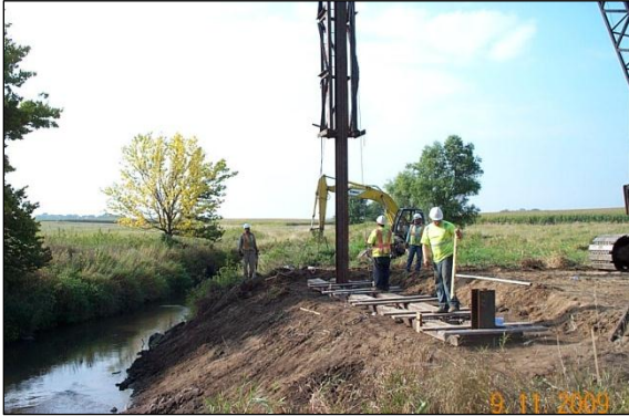
c. Pile driving in west abutment
