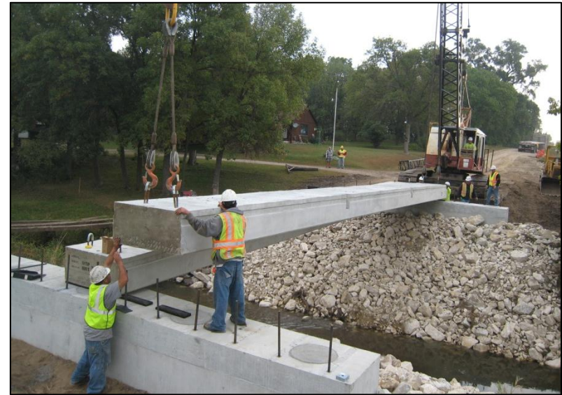
d. Setting of Beam #5
