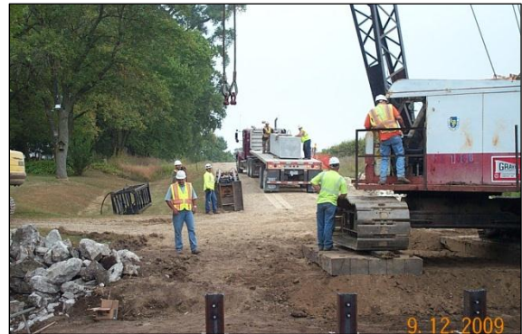
f. East abutment cap arriving at site
