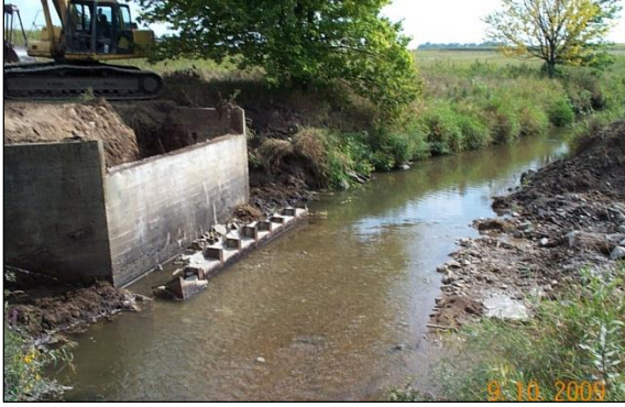
a. Existing east abutment
