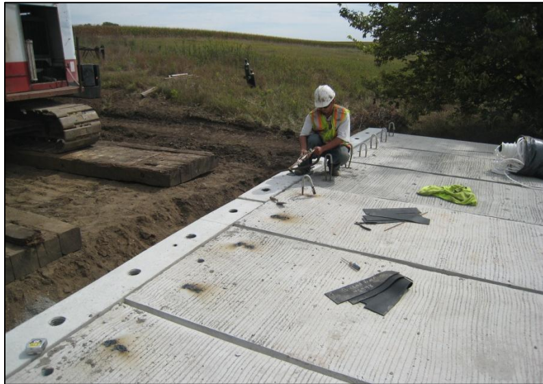
k. Cutting off beam lift cables
