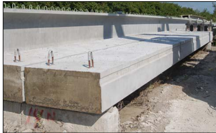
Figure 2.14. Voided precast beams
