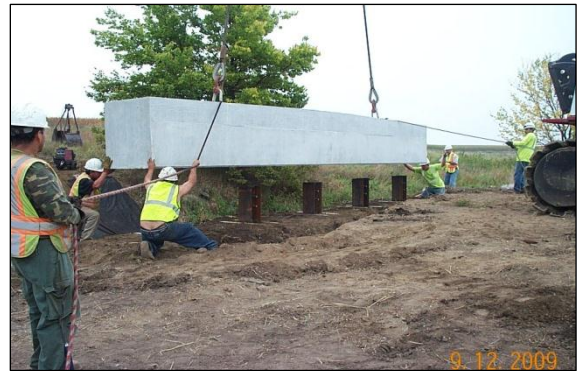
h. Installing west abutment cap
