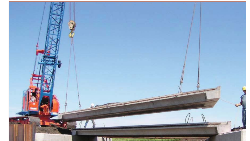
Using a crane to position a precast deck panel at the Mt. Vernon Road Bridge in Black Hawk County
