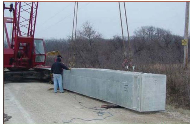
Precast abutment cap at Madison County bridge site
