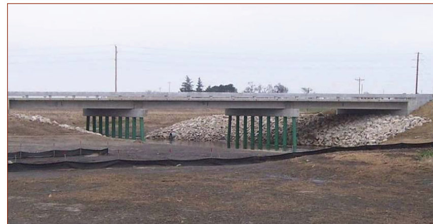
Completed bridge over 120th Street, Boone County
