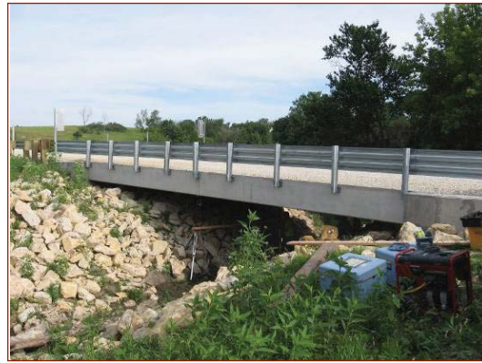
Completed box girder bridge in Madison County
