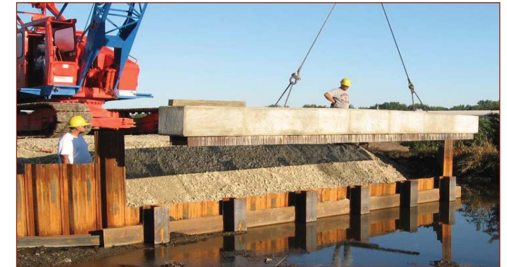
Placing a precast concrete abutment cap
