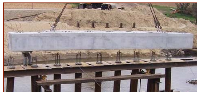
Precast pier cap lowered into place at Boone County bridge site
