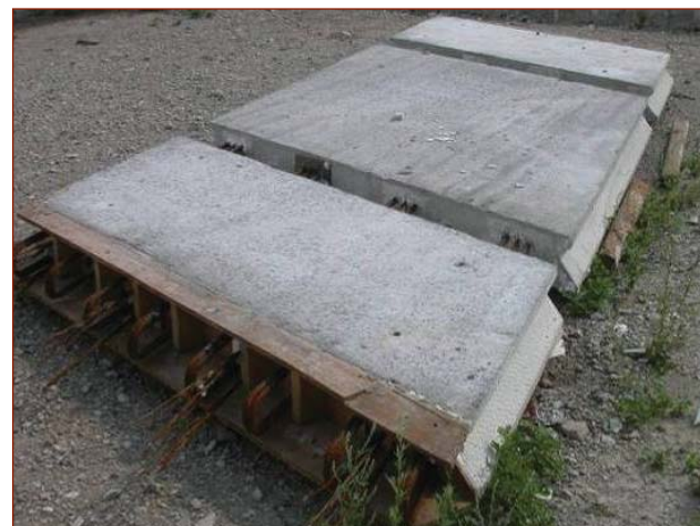
Full-depth precast concrete bridge deck panel used in the Boone County bridge
