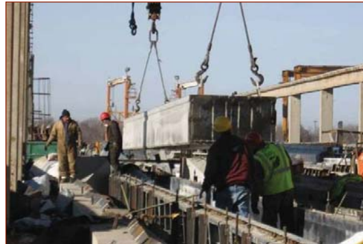
Fabrication of a precast box girder for the Madison County bridge
