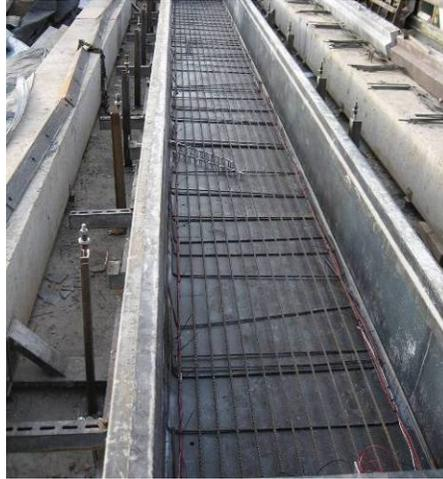
**Figure 2.7. Photograph of box girder form with bottom pretension strands**
