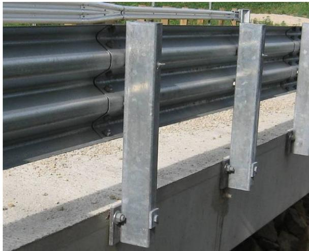
**Figure 2.4. Photograph of bridge guardrail system**
