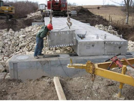
**c. placing girder into final position**
