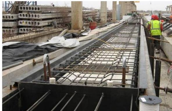
**Figure 2.8. Photograph of top of beam reinforcing and foam core**
