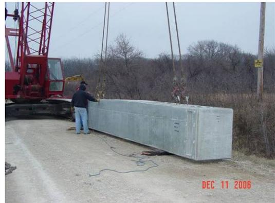
**b. lifting of precast abutment cap**
