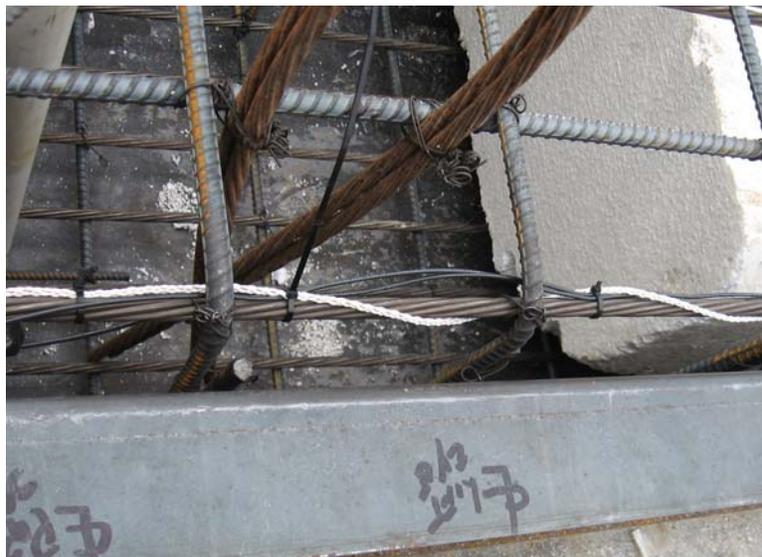
**Figure 6.17. Corrosion electrode wrapped around strand**
