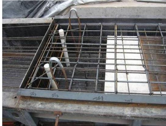
**Figure 2.9. Photograph of end reinforcing and lift points**
