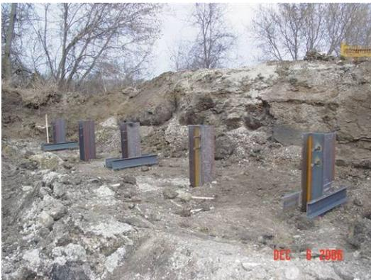
**a. finished installation of steel piles**
