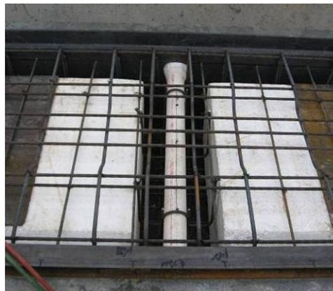
**Figure 2.10. Photograph of midspan transverse tie duct**
