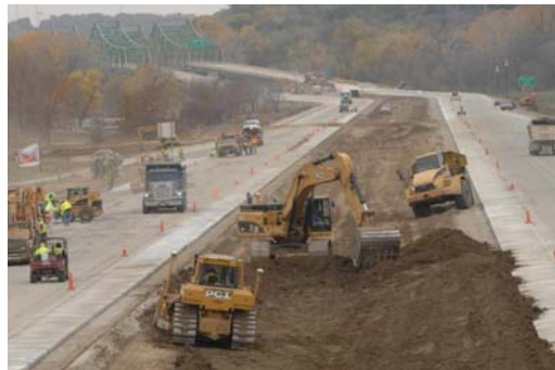
I-680 construction leading to Memorial Bridge. Photo by Iowa DOT.
