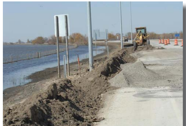
I-29 near Hamburg, taken during construction on Oct. 5, 2011. Photo: Iowa DOT
