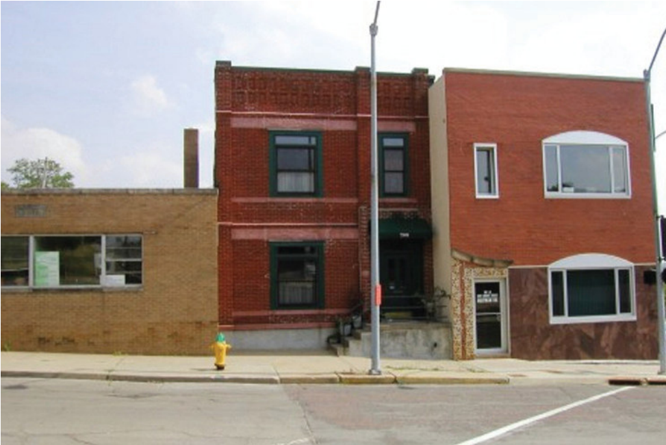
711, 709 and 707 E. Locust (left to right). 711 has already been removed. 709 and 707 will be moved or demolished so the West Capitol Terrace can be completed.
