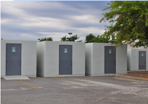
Joplin, Mo., Aug. 15, 2011 – The safe rooms at the temporary Joplin High School. The EF-5 tornado on May 22, 2011, tore a path through Joplin seven miles long and half a mile wide. Photo by Elissa Jun/FEMA.
