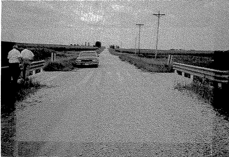
a. Overall view
