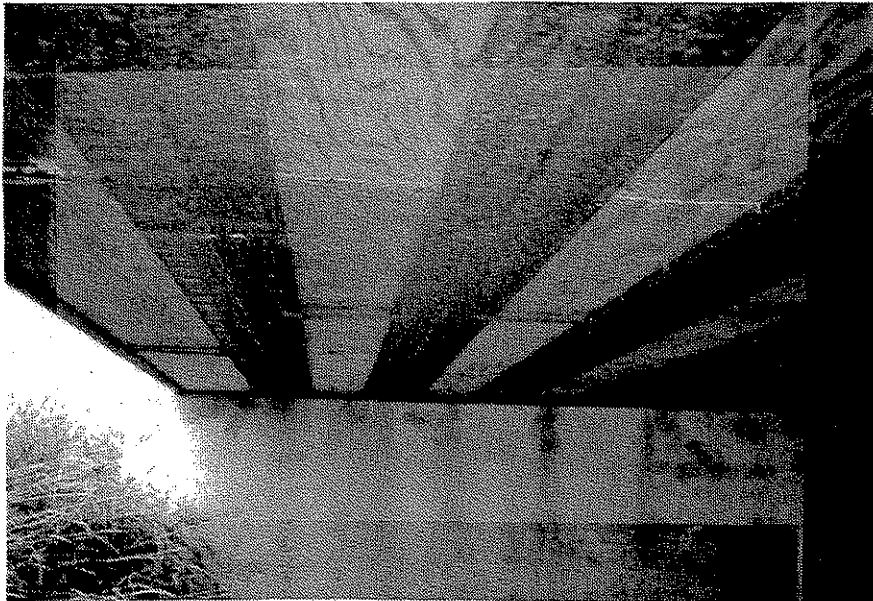
b. Plywood forms in place
