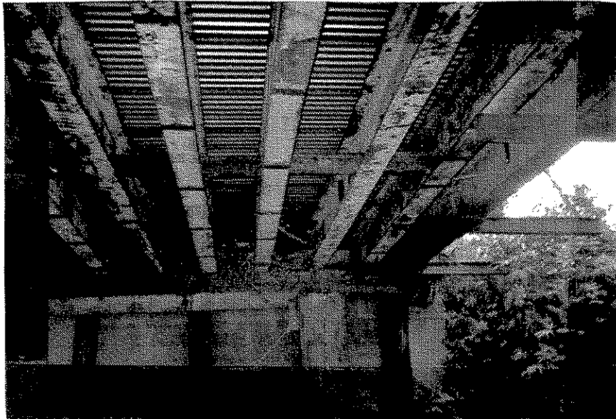
b. View showing metal decking
