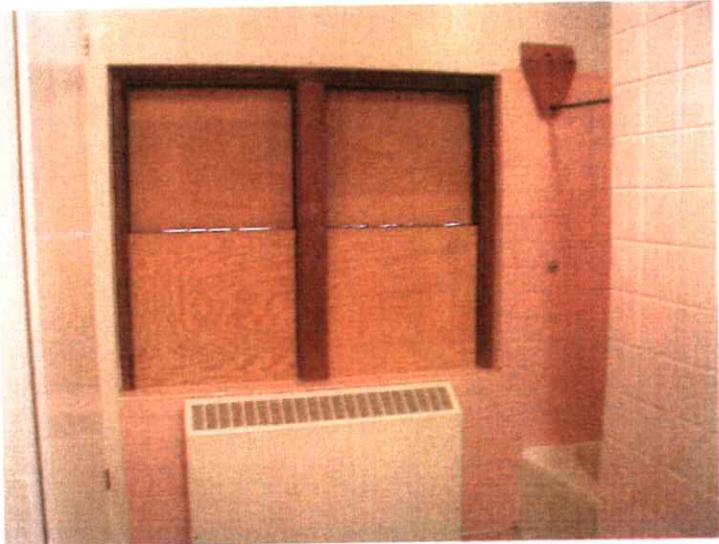
• Windows boarded up for safety of youth
