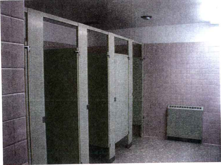
• No urinals in boys' living unit • Partitions are corroded
