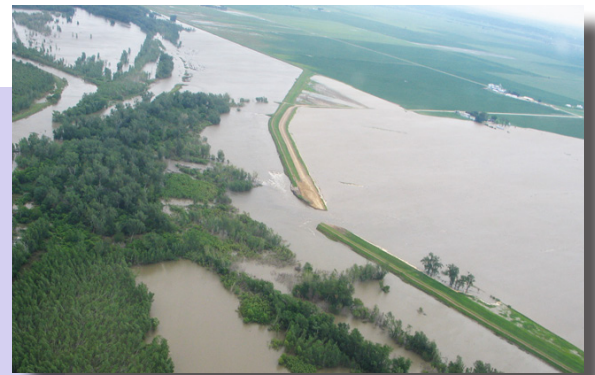
June 13 - Breached levee near Hamburg, Iowa. Photo by the Iowa Dept. of Public Safety.
