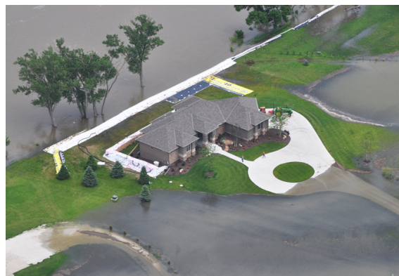
June 24 – A home along the Missouri River is nearly completely inundated by flood waters. Photo by Iowa National Guard.
