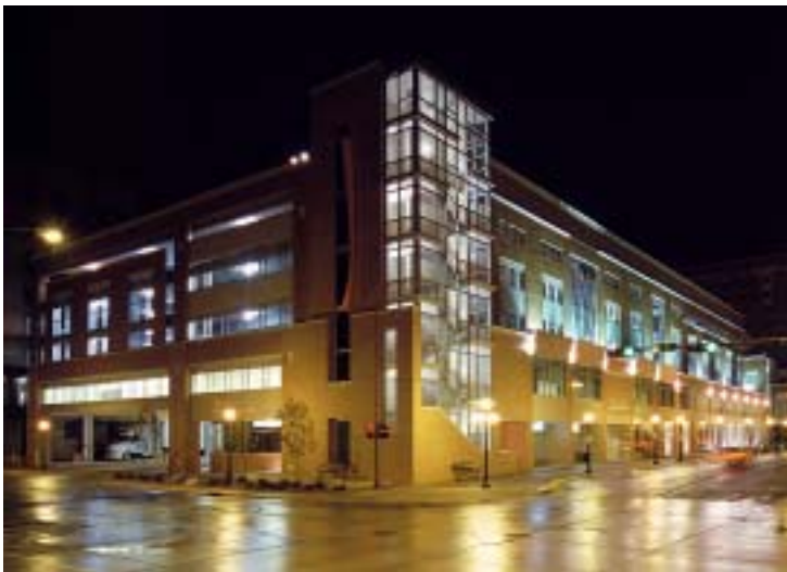
Sioux City's new Martin Luther King, Jr., Transportation Center
