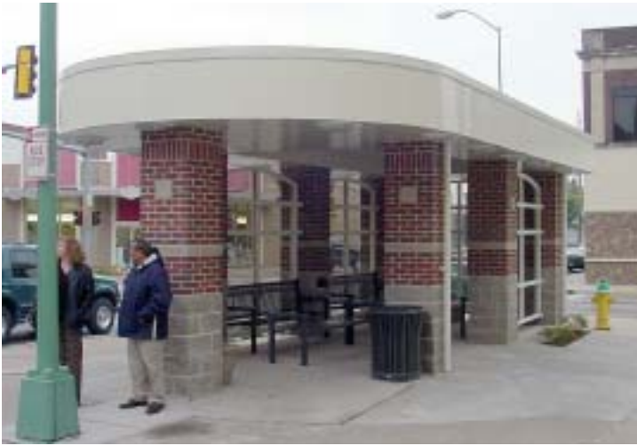
Ottumwa Bus Passenger Transfer Station
