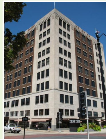
Renovated Roshek Building, home of IBM Dubuque offices. Source: City of Dubuque
