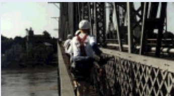
The Katy Trail features many historic railroad bridges.
