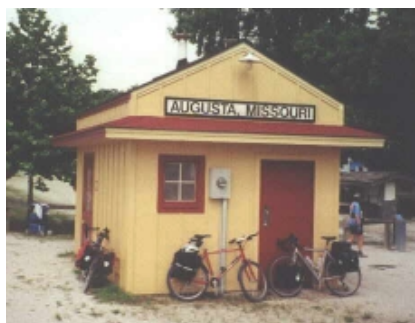
By providing public services to users of the Katy Trail, the town of Augusta, Missouri has established itself as a trail-friendly community. This attractive historic building was refitted for public restrooms for trail users.
