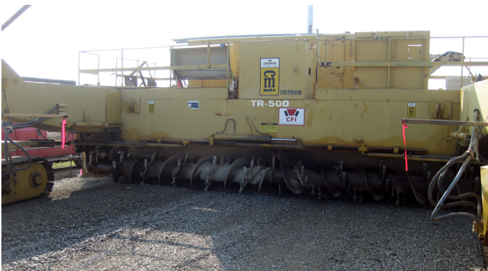
Figure 10 – On-site conditions and construction operations
