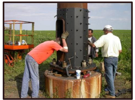
A bolted reinforcing jacket was placed on a tower in the I-35 & US 18 Interchange near Clear Lake
