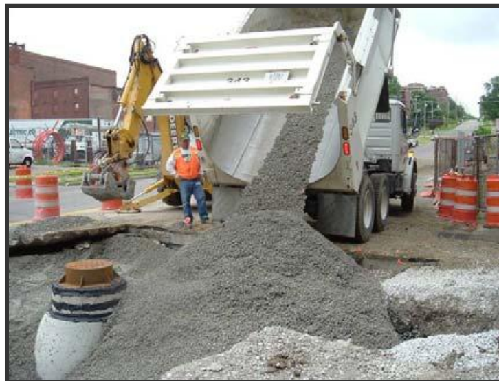
Large lift thickness used in utility cut trench backfilling
