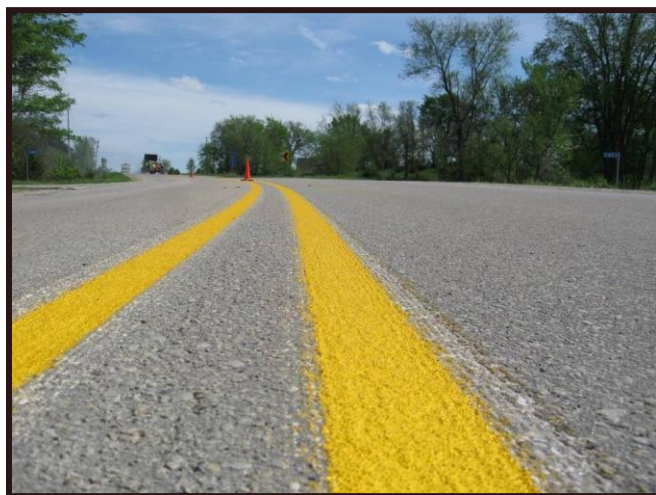
A pavement marking test deck in Dallas County, evaluating experimental centerline markings placed within a groove.
